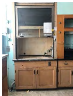
Figure 1. Older fume hood without automatic sash
