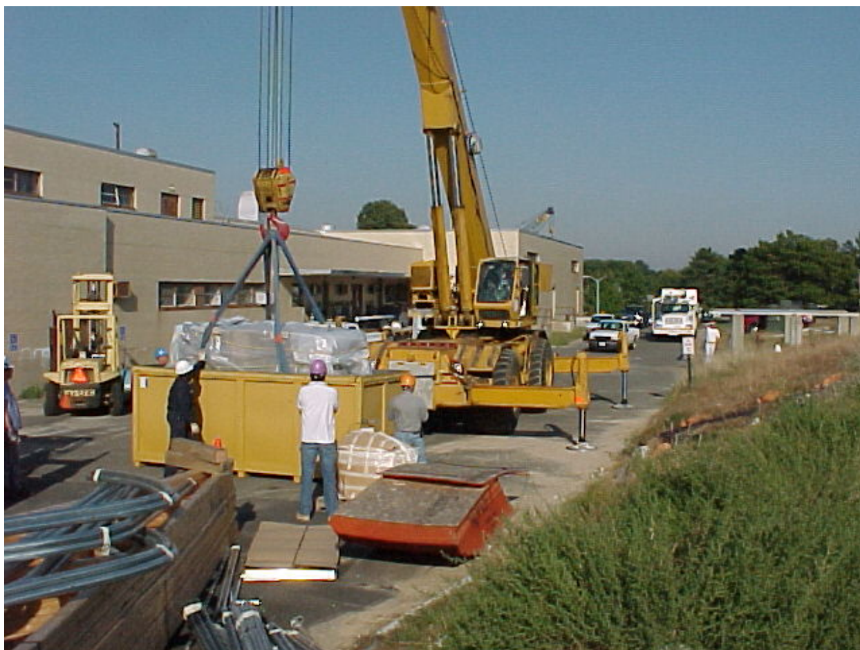
A portable 70-ton crane was used to move the East Yard Sump and place it into a disposal container.
