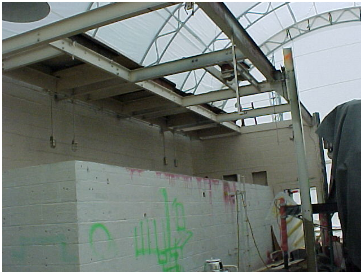
The Water Treatment House looking east with the concrete roof panels partially removed. The Canal House has been removed; it used to be on the right side of the picture. Green paint was used to demarcate de-energized electrical equipment that was removed from the wall.
