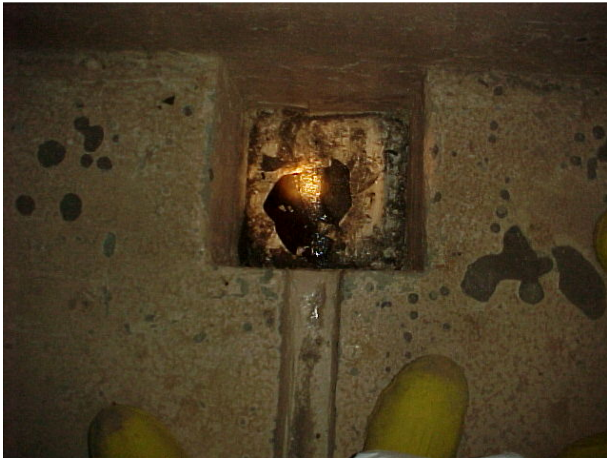
One of the Canal's three floor low-point drain sumps. A flashlight supplied the source of light for this picture; hence, the odd glow in the bottom of the sump. Note the paint peeling from the surrounding floor surfaces. The sumps were removed.
