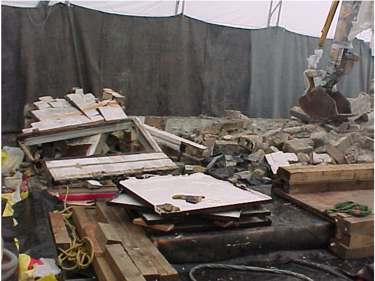
A small portion of the debris from the wreckage of the Water Treatment House. Such material was loaded into B-52 containers for disposal at a licensed offsite facility.
