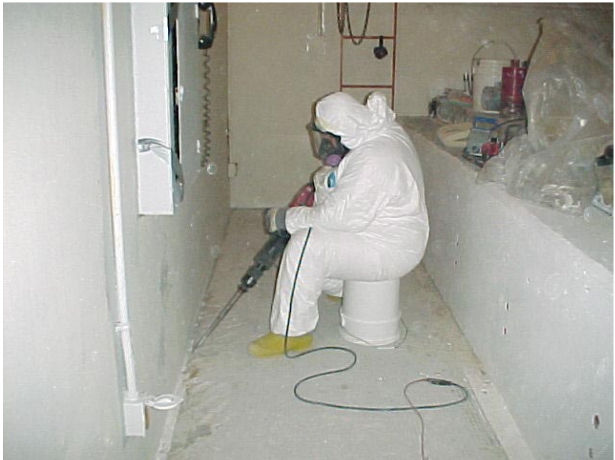
A worker is using an electric chipping hammer to remove the contamination from the corners where the walls and floor meet.
