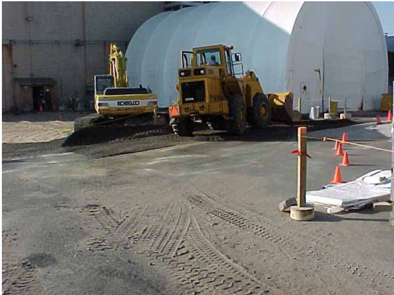
Fill being placed into the area to allow vehicles' access to the west truck-bay door of Building 801 so as not to affect Laboratory operations in that building.
