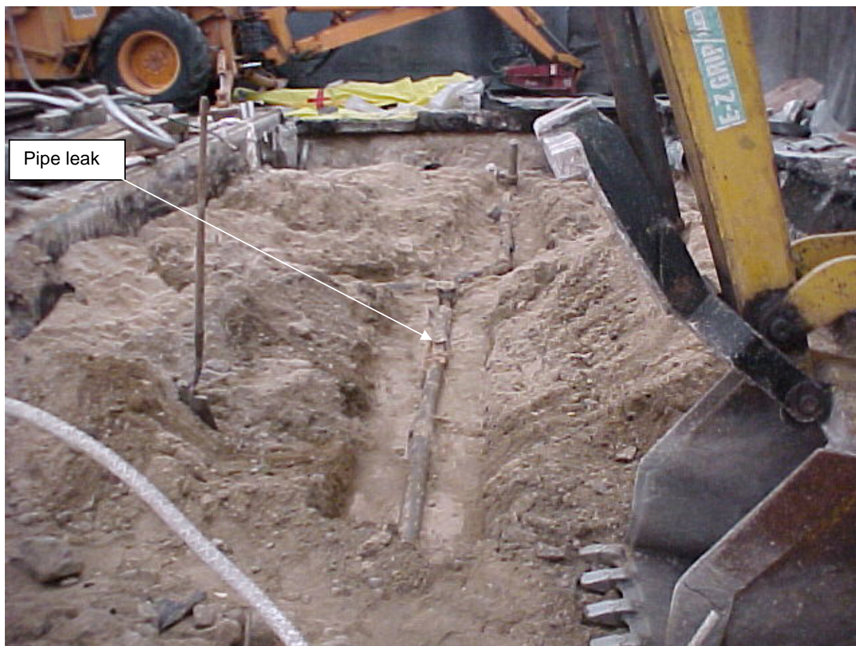
The Water Treatment House's floor drain system looking west, towards Building 701. Just west of the first drain, the pipe leaked water contaminated with Cs-137 and Sr-90 to the soil.
