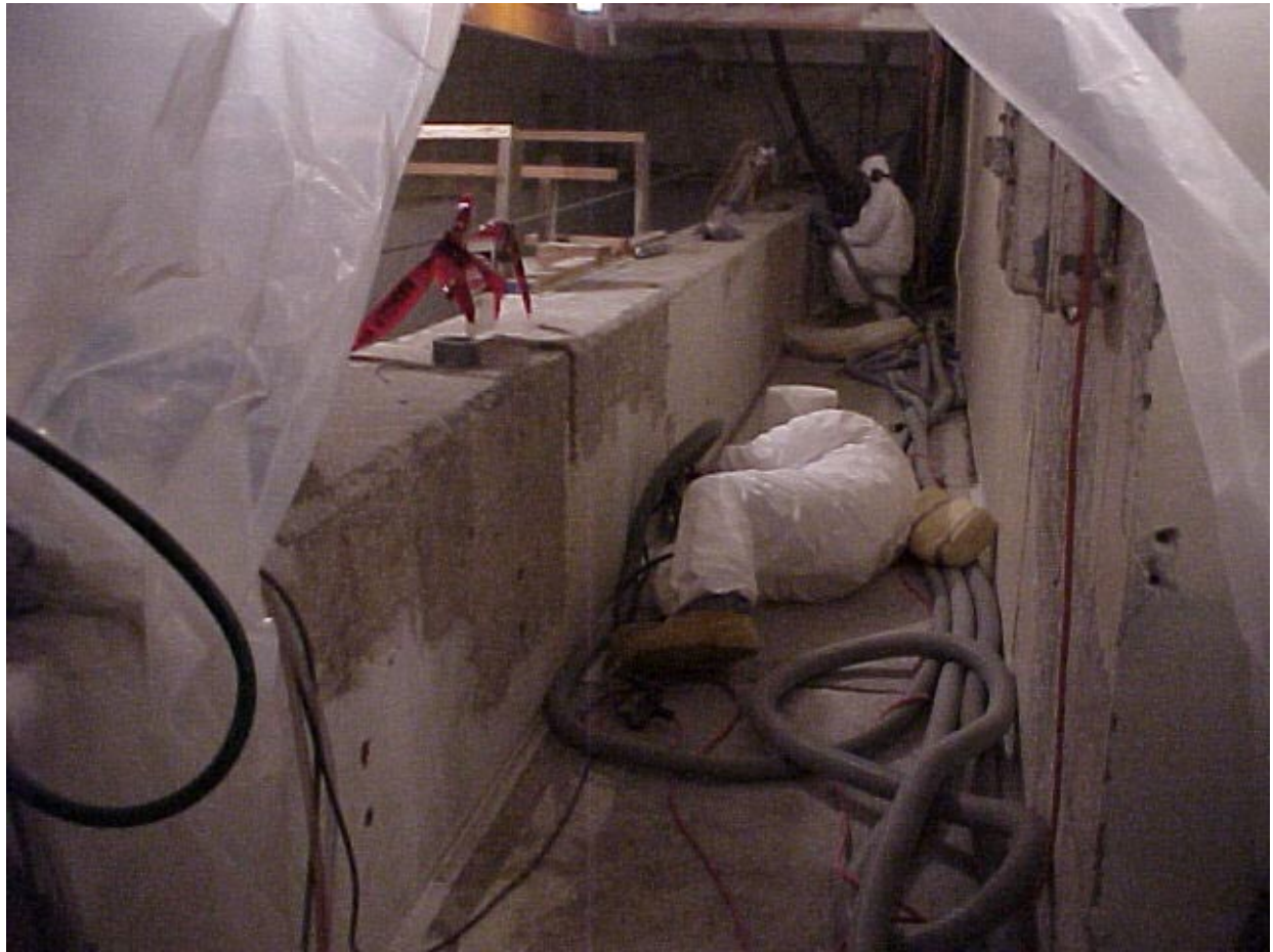
Workers using hand held scabbling equipment to clean the walls of the Canal's walkway. The workers wear protective clothing and use respirators.
