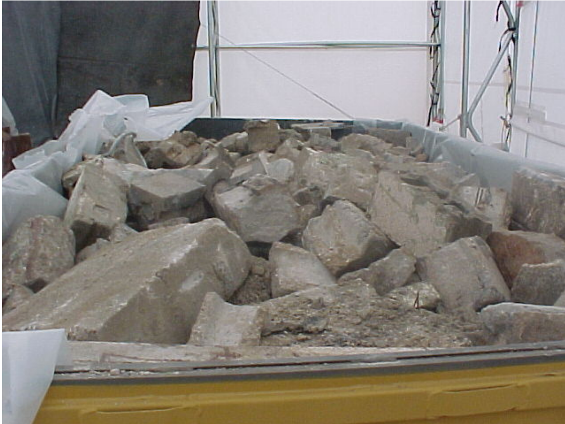
B-52 box filled with concrete debris from demolishing of the Water Treatment House.
