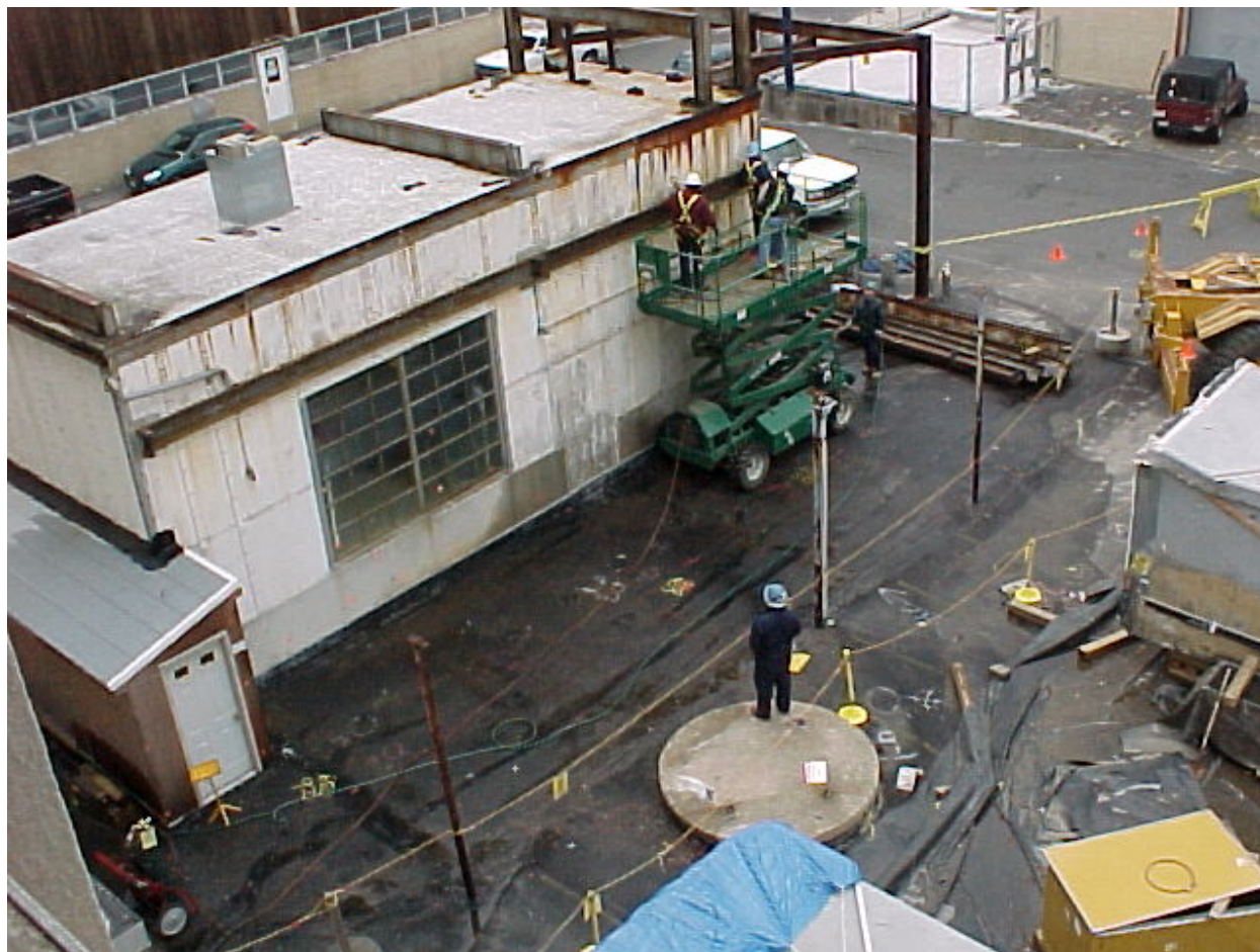
Looking northeast from Building 701, the steel awning superstructure being removed from the south side of the Canal House.
