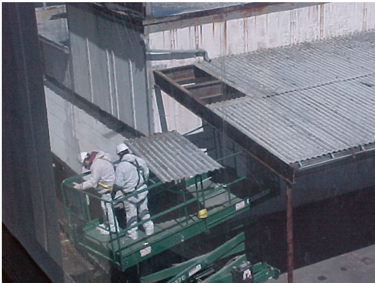
Asbestos workers on a manlift, removing awning panels. Each panel contained asbestos, requiring piece-by-piece removal, rather than allowing the material to fall and shatter.
