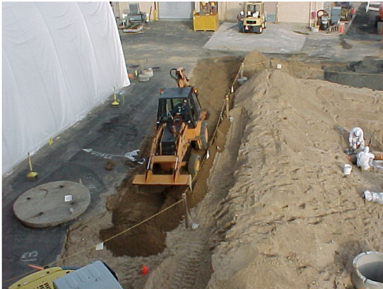
Back fill of the area near the south side of the large tent. A lift then was placed in this area to assist in the disassembling of the large tent.
