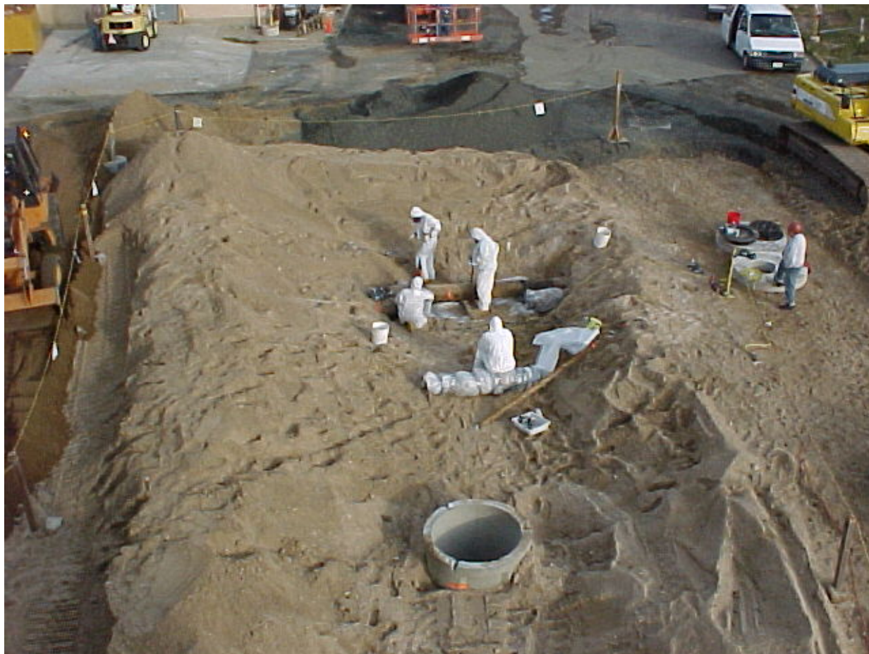
Looking east, of the abandoned chilled-water and air lines are moved from the new storm drain trench. Workers were protective clothing and respirators due to the pipes' asbestos coating and the potential for the piping to be internally contaminated. One of the new storm drain catch basins has been installed near the bottom of the picture.
