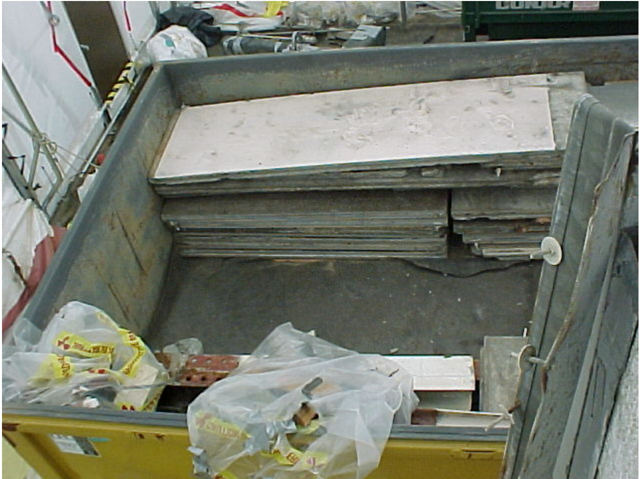
Asbestos-containing roof slabs were packaged for disposal.
