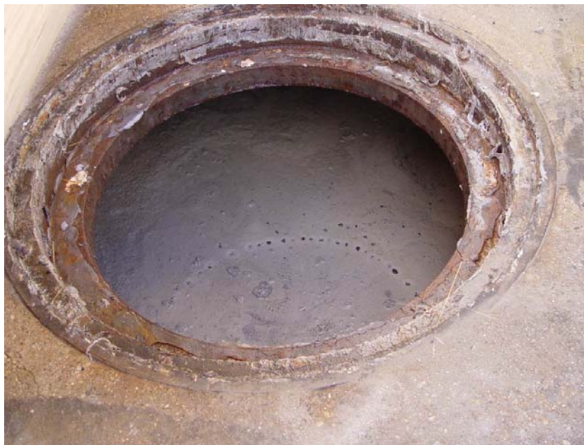
Photograph 7 – Grouted South Side Building 701 Air Plenum
