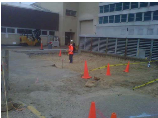
Photograph 10 – Performing as-left radiological walkover survey prior to installation of the engineered cap
