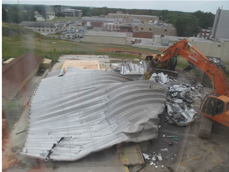
Photograph 2 – Demolition of the DSB
