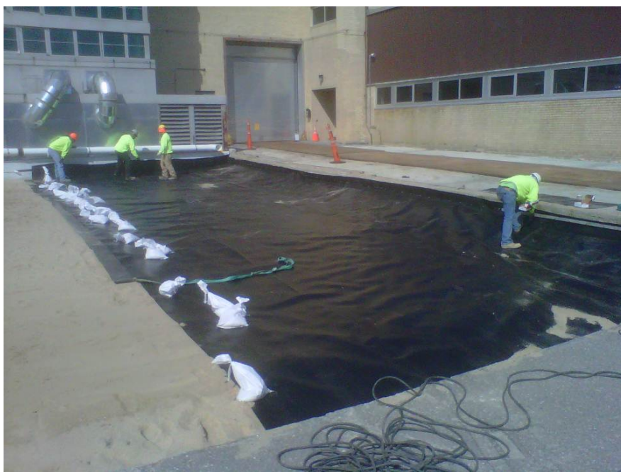
Photograph 12 – Installation the HDPE liner near the Building 701 east rollup door
