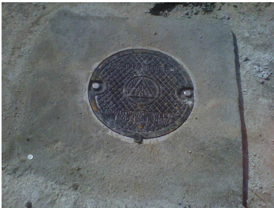
Photograph 18 – Finished flush-mount groundwater monitoring well.
