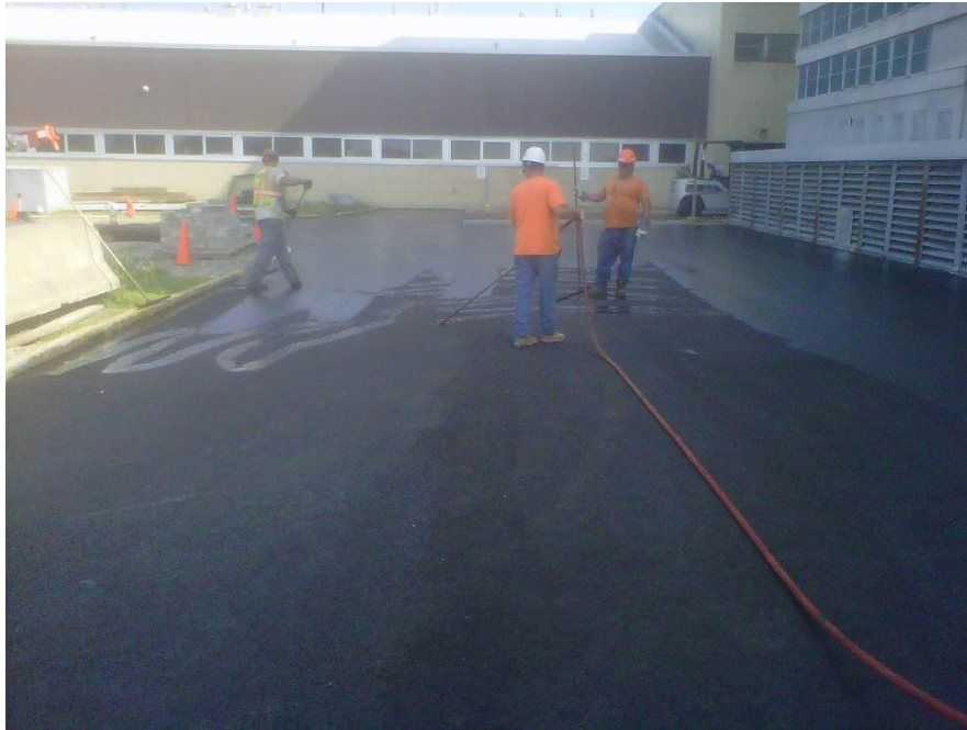
Photograph 16 – Treating asphalt surface with seal coat west of Building 701
