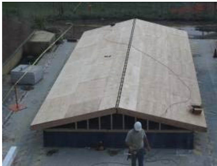
Photograph 3 – Installation of the permanent roof over the BGD filter opening
