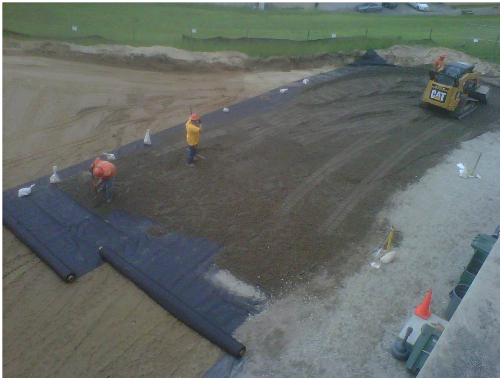
Photograph 15 – Installation of crushed stone protection layer
