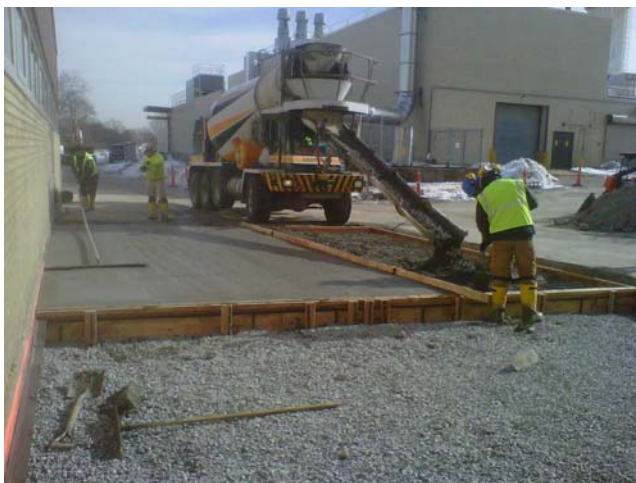
Photograph 11 – Installation of the concrete pad near the Building 701 east rollup door.
