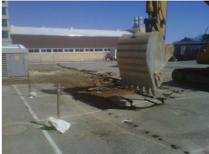
Photograph 8 – Removal of existing asphalt
