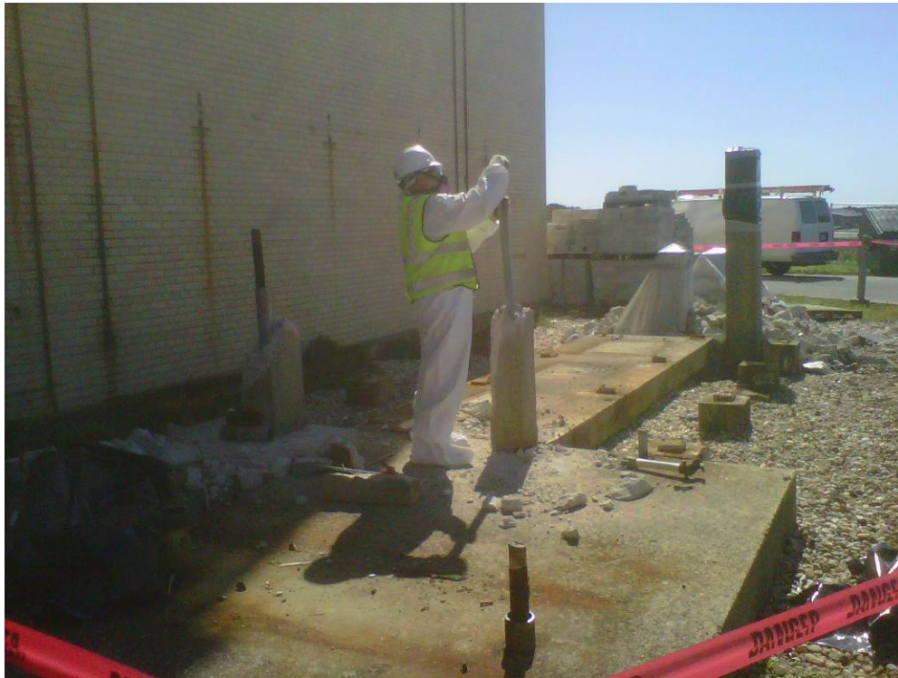
Photograph 6 – Asbestos abatement at previous location of Building 701 transformers
