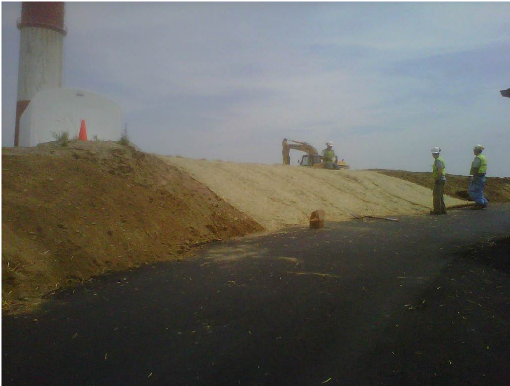
Photograph 19 – Installation of erosion controls along eastern border of finished engineered cap.
