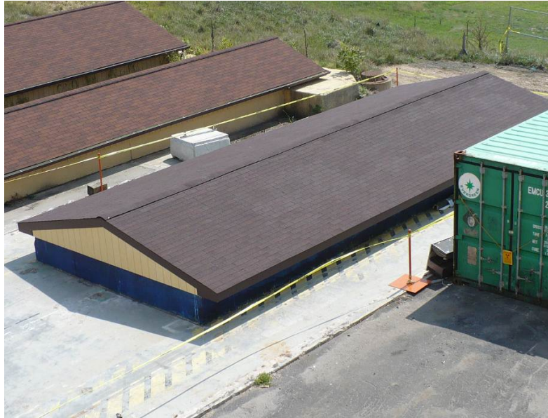
Photograph 4 – Completed permanent roof over BGD filter opening
