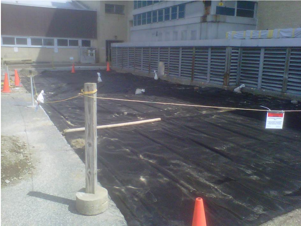
Photograph 14 – Geotextile layer installed west of Building 701
