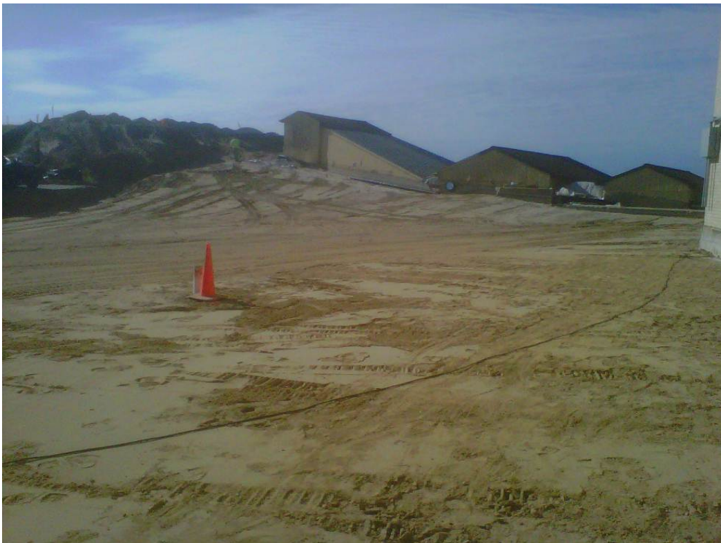
Photograph 13 – Area south of Building 701 after placement of 12-inch sand protection layer
