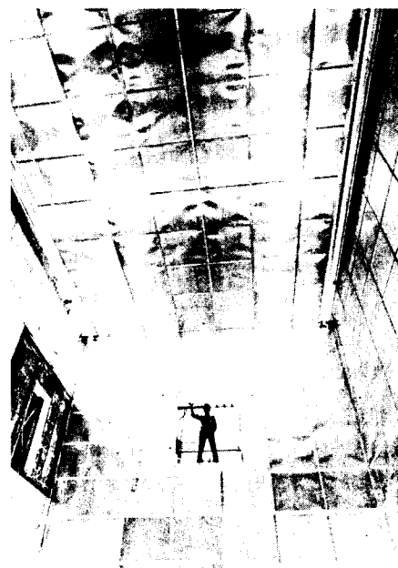
A completely shielded room has been constructed to house the Cockcroft-Walton injector for the new Linac of the Alternating Gradient Synchrotron. In this shielded room the particles will originate that eventually reach a speed of 99.9% the speed of light before striking a target.
