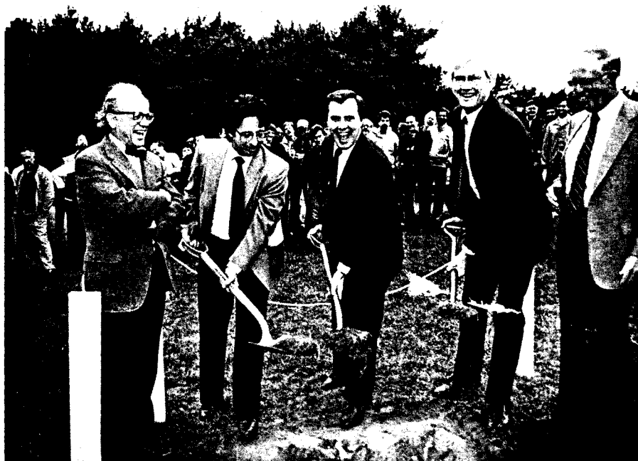
The first three spadeful of earth for the beam transfer line were moved by (from left) Nicholas Samios, William Carney and Alvin Trivelpiece. Carney wielded the spade which broke the ground for the AGS, Trivelpiece the shovel originally enlisted for the groundbreaking for the Tandem, and Samios a new spade, befitting the new project. After Herman Feshbach (left), Robert Hughes (right), and other guests took their turns at digging the tunnel, the employees attending the ceremony were all invited to follow suit.
