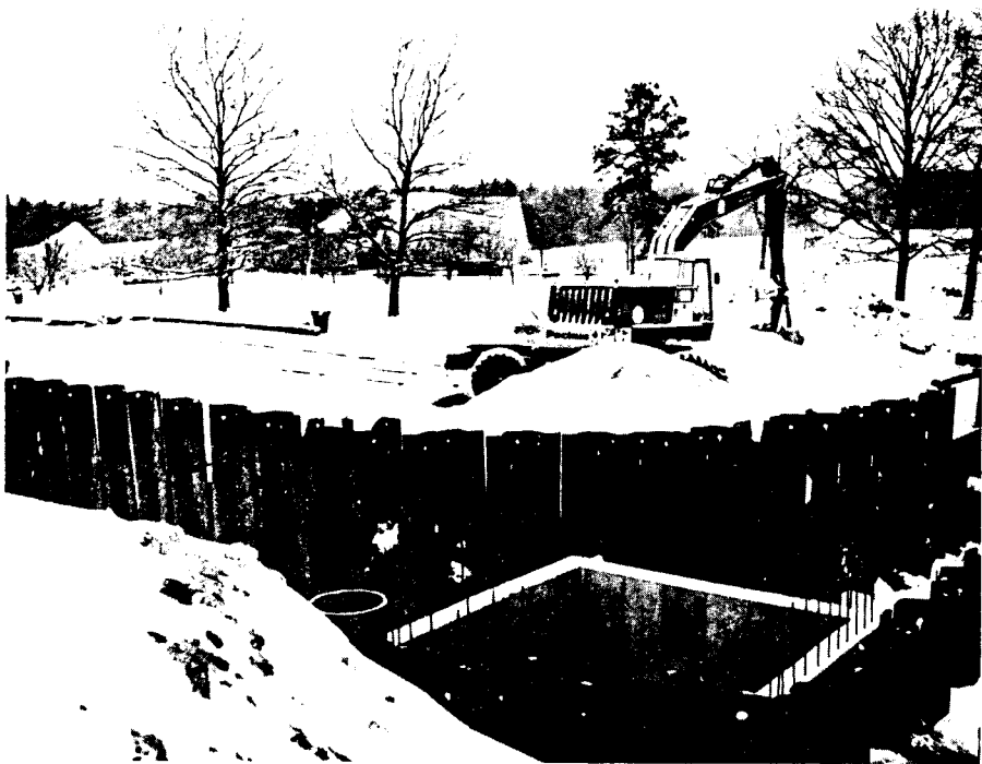
The year ended with detours, when, in November, excavation began to provide central steam and sewage service to the new firehouse, which is being constructed on the northwest corner of Upton Road and Brookhaven Avenue. At the time of the first snowfall in late December, work was well under way.
