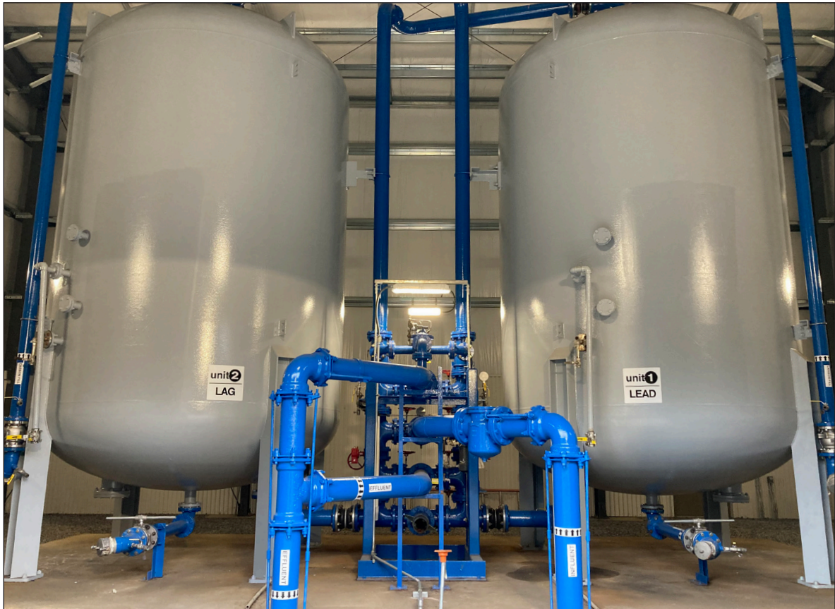
Granular Activated Carbon Filter Vessels at Former Firehouse Groundwater Treatment System Building
