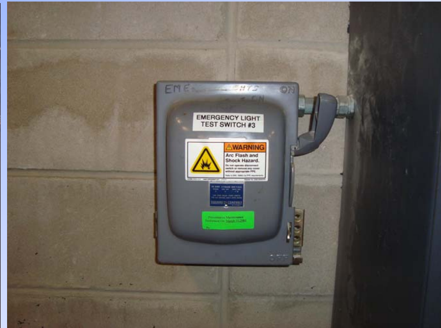
208V < 225A Disconnect Switch
