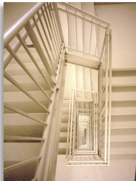
This stair enclosure is provided with a continuous tubular metal handrail to help occupants navigate the stairs safely.
