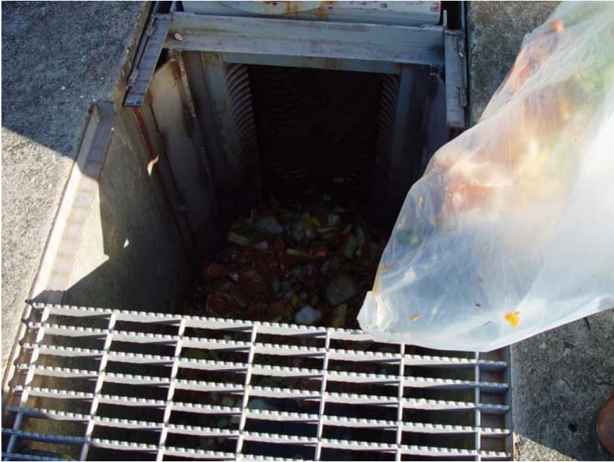
Figures 1-3. Sewage Treatment Plant operator feeding cafeteria food scraps into the head of the plant.
