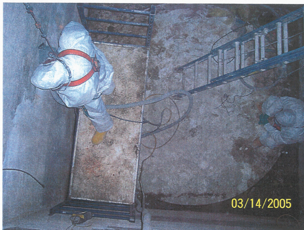
Photo 14: Use of a HEPA vacuum was required during scabbling activities to reduce potential hazard of airborne contaminants
