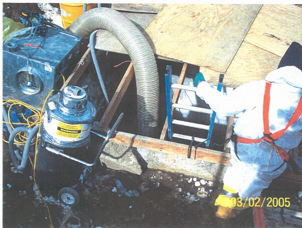
Photo 14: Use of a HEPA vacuum was required during scabbling activities to reduce potential hazard of airborne contaminants
