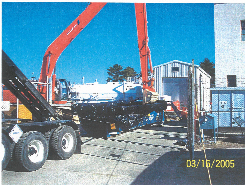
Photo 10: Soils from the D Yard were loaded directly into lined roll-off containers
