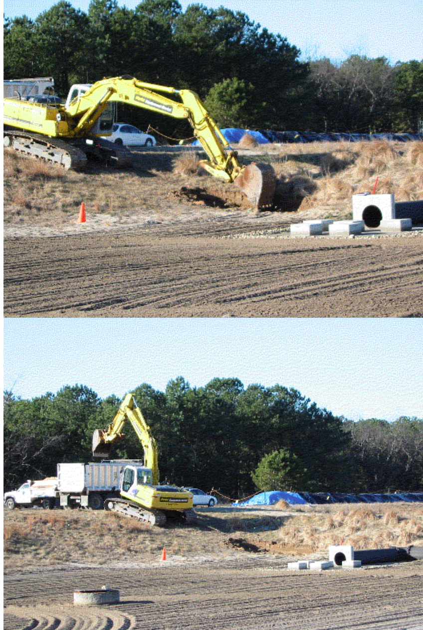
Photograph : Track excavator removing soil from STP sand filter bed/berm and loading a dump truck for transport to the soil pile storage area (in background).
