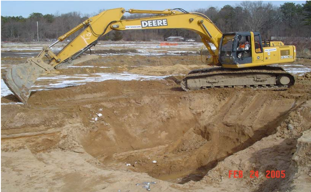
Photograph 1 – Soil removal at the former HWMF.
