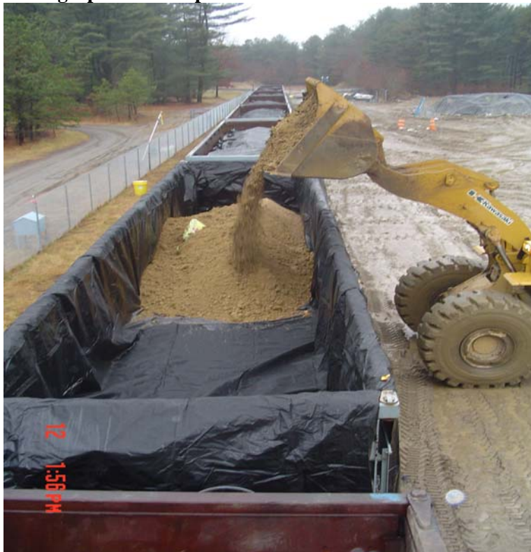
Photograph 8 – Loading railcars with waste soil at the former HWMF.
