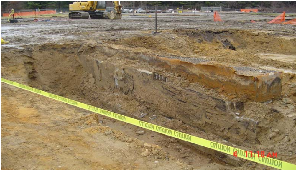
Photograph 6 – Discovered sub-surface structure as the former HWMF.
