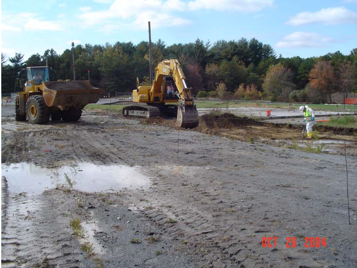
Photograph 2 – Excavating and surveying at the former HWMF.
