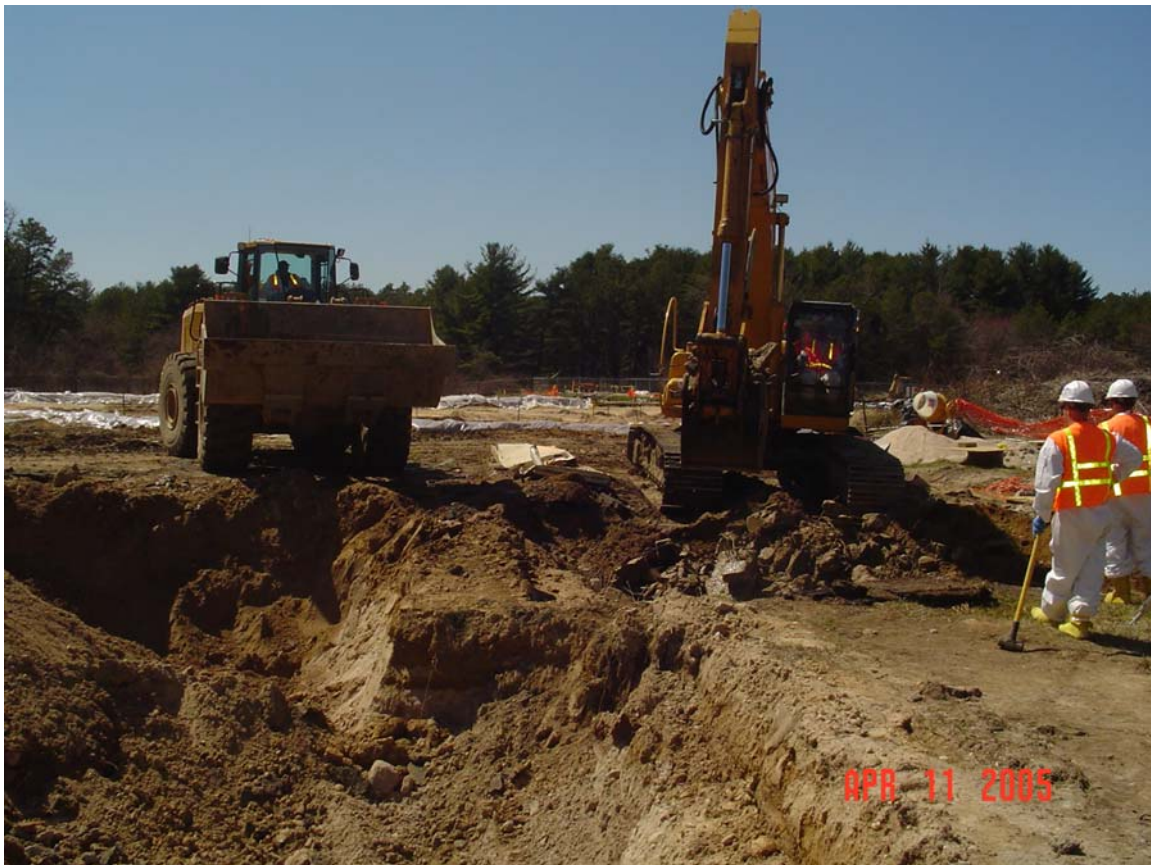
Photograph 3 – Uncovering trench at the former HWMF.
