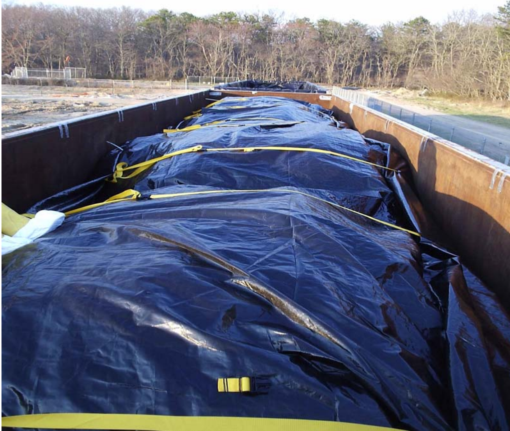
Photograph 9 – Sealed Black Stallion® liner in railcar at the former HWMF.
