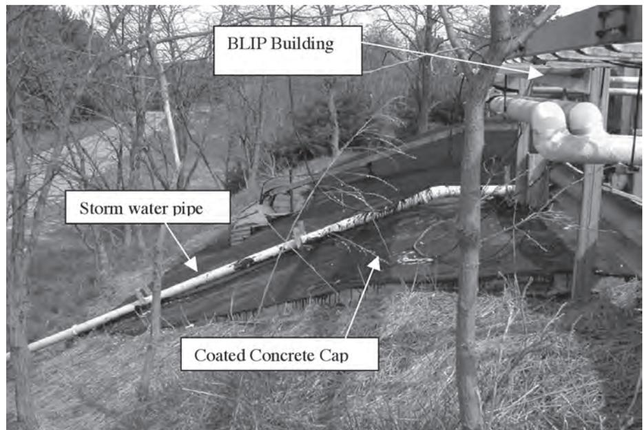
FIGURE 6. Concrete cap on the west side of the BLIP facility. White pipe conveys stormwater collected from roof drains away from the building.
