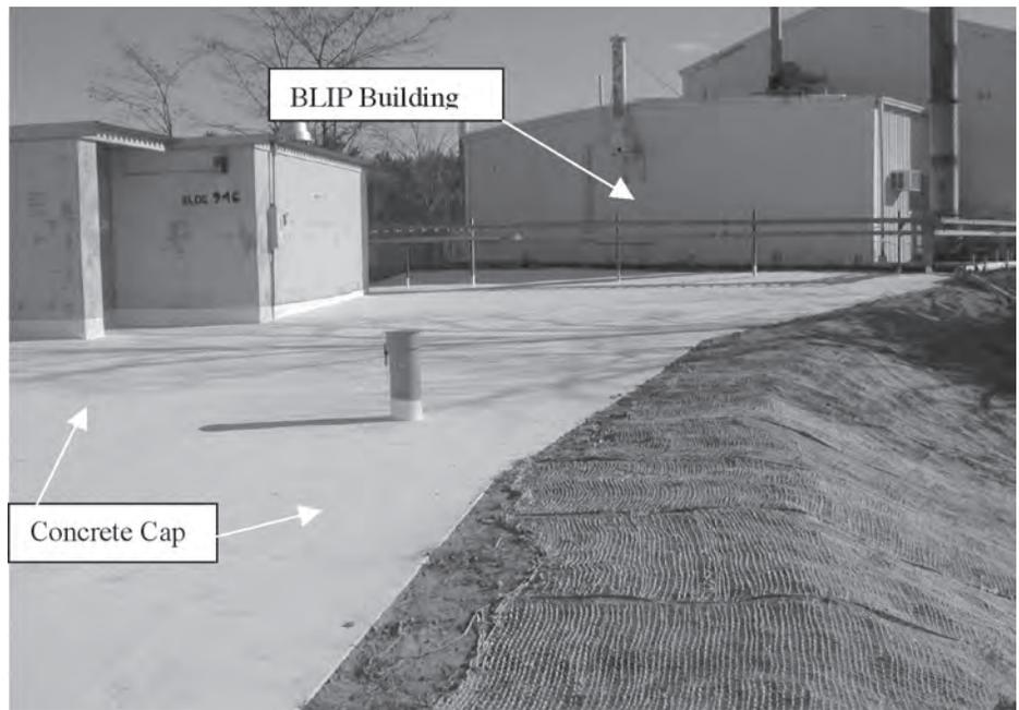
FIGURE 5. Concrete cap on the north side of the BLIP facility. Pipe is an upgradient monitoring well.
