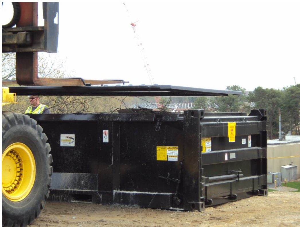
Photograph 7 – Packaging project waste in intermodal shipment container
