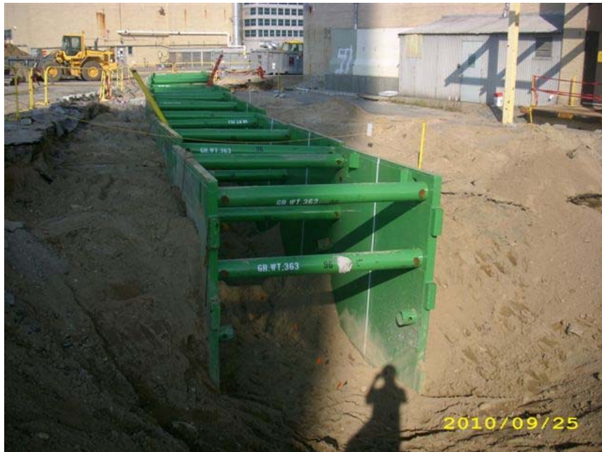
Photograph 4 – Trench boxes installed in Phase III, Trench 4
