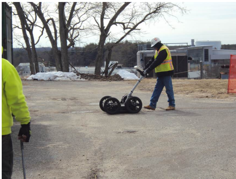
Photograph 1 – Marking out utilities with ground-penetrating radar prior to excavation
