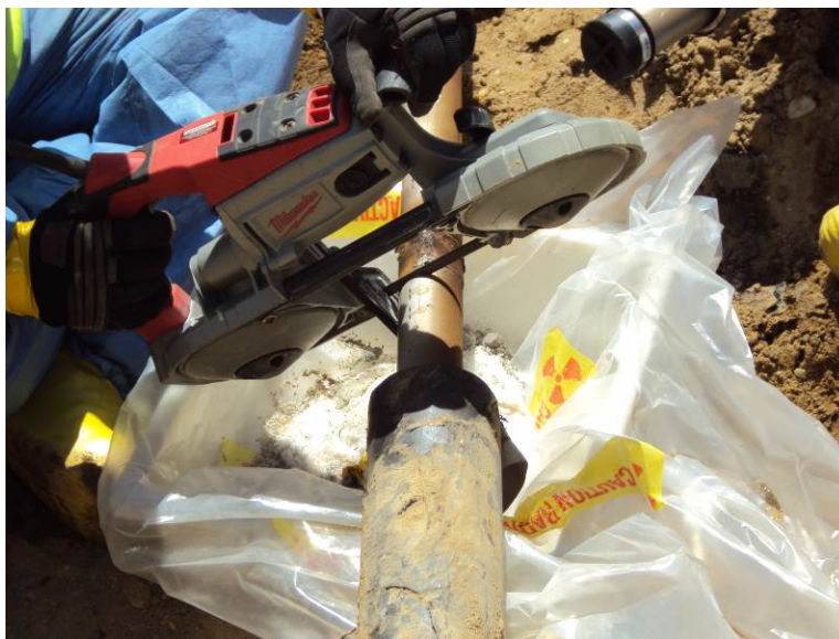
Photograph 3 – Cutting 2-inch stainless steel inner D/F Waste Line
