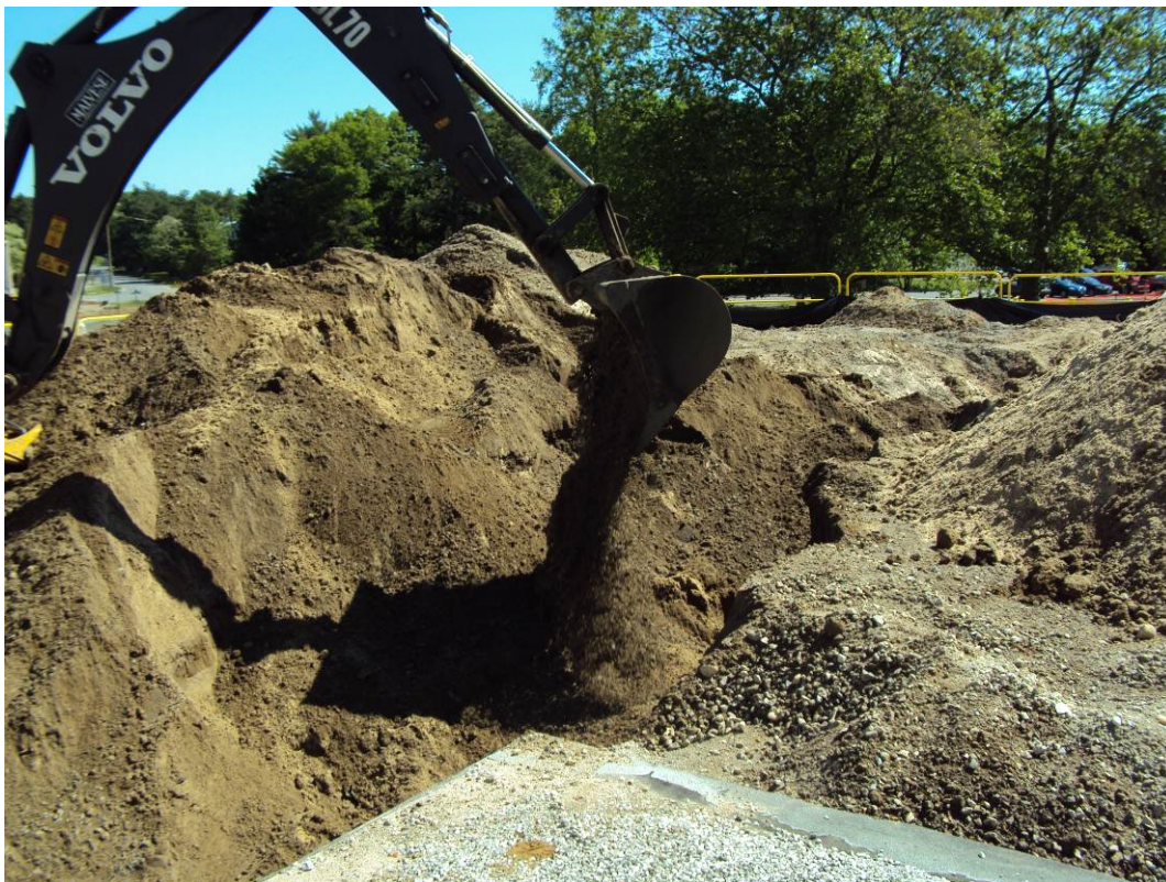
Photograph 8 – Backfilling Phase II Trench
