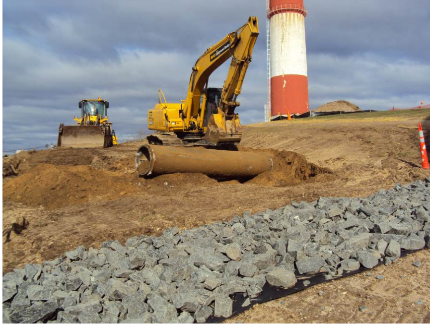
Photograph 2 – Removal of 30-inch duct during Phase I of the project
