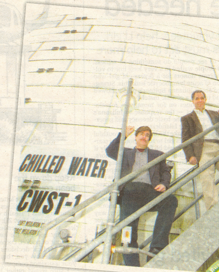
Mark Toscano (left) and Peter Pohlot climb the stairs of Brookhaven National Laboratory's 71-foot chilled water facility, which has reduced electric demand by 2,000 kilowatts during peak daytime periods, saving over $2 million in energy costs since 1998.
