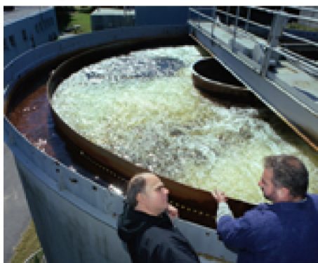
3. AERATION TANK reduces carbon dioxide gas and aids in the oxidation of iron. At the aeration tank, Steve Barcelo (right) describes the action to Frank Masia.
