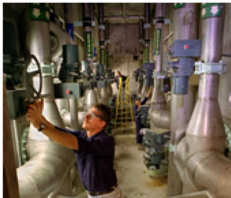
7. FILTRATION is performed, using what is called a rapid sand filter made up of eight filter cells containing sand and anthracite coal. Inspecting the valves in the filtration valve gallery are: (front to back) Jack Kulesa, Richard Lutz, and Steve Barcelo.
