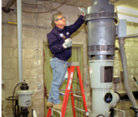
1A. WELLS 4, 6, and 7 provide source water high in iron that must be "finished" at BNL's Water Treatment Facility (WTF). At one of these wells, Phil Pizzo performs preventive maintenance on pump motor.
