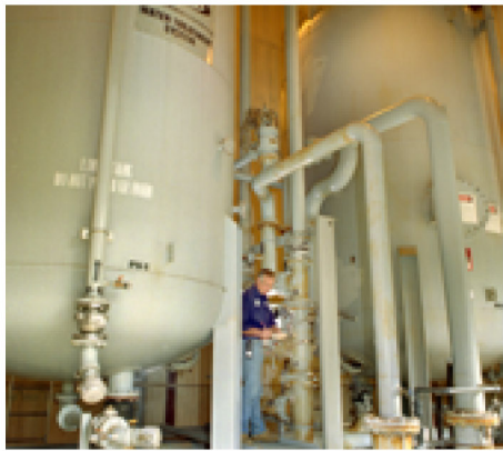
1B. CARBON FILTRATION AT WELLS 10, 11, and 12 is designed to remove volatile organic compounds before the low-iron water from these three wells directly enters the drinking-water distribution system. Noting the pressure of the carbon filtration system is Richard Lutz.
