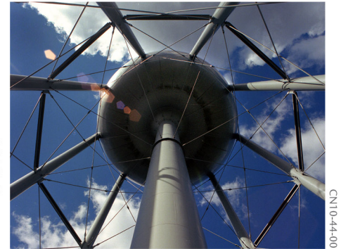
12. ONE-MILLION-GALLON WATER STORAGE TOWER , as viewed from its base, is the larger of the Lab's two water towers. Built in 1985, and located at Cornell and North Sixth Street, this tank is 126 feet above the ground; its bowl is 75.5 feet in diameter. Located next to Police Headquarters, Bldg. 50, the other water storage tank holds 300,000 gallons and was built for the U.S. Army in 1941, when the site was Camp Upton. Water from the two towers is delivered on site at a pressure of 55 to 70 pounds per square inch via 45 miles of distribution pipe. The piping is a mix of cast iron dating from World War II Camp Upton, transite, plastic, and cement-lined ductile iron. When pipe is added or replaced, cement-line ductile iron is used.
