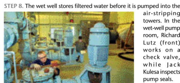
**STEP 8.** The wet well stores filtered water before it is pumped into the air-stripping towers. In the wet-well pump room, Richard Lutz (front) works on a check valve, while Jack Kulesa inspects pump seals. — CN10-38-00
