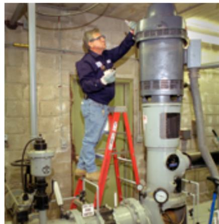
**STEP 1A.** Wells 4, 6, and 7 provide high-iron source water which must be "finished" at BNL's Water Treatment Facility (WTF). At one of these wells, Phil Pizzo performs preventive maintenance on a pump motor. — CN10-144-00
