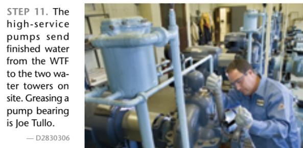
**STEP 11.** The high-service pumps send finished water from the WTF to the two water towers on site. Greasing a pump bearing is Joe Tullo. — D2830306
