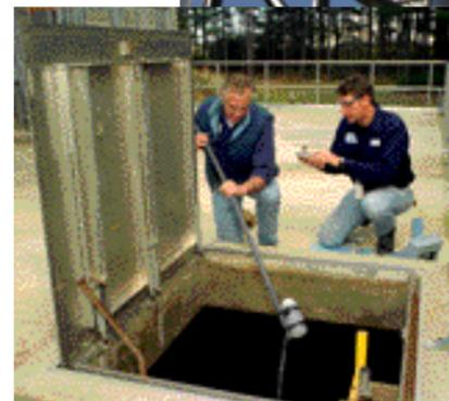
**STEP 10.** At the clear well, where up to 250,000 gallons of "finished" water is stored before its final chlorination and distribution, Richard Lutz and Jack Kulesa take samples. — CN10-146-00
