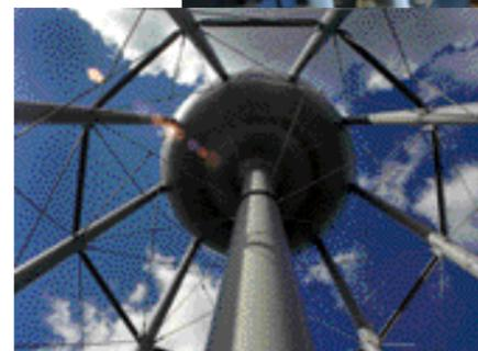
**STEP 12.** Water from the Lab's two storage towers is delivered on site at 55 to 70 pounds of pressure per square inch via 45 miles of distribution pipe. Viewed from its base is the larger of the Lab's towers, which holds one million gallons of water. — CN10-44-00
