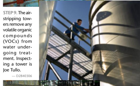
**STEP 9.** The air-stripping towers remove any volatile organic compounds (VOCs) from water undergoing treatment. Inspecting a tower is Joe Tullo. — D2840306
