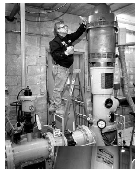
STEP 1A. Wells 4, 6, and 7 provide high-iron source water which must be "finished" at BNL's Water Treatment Facility (WTF). At one of these wells, Phil Pizzo performs preventive maintenance on a pump motor. — CN10-144-00
