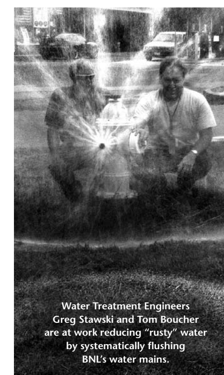
Water Treatment Engineers Greg Stawski and Tom Boucher are at work reducing "rusty" water by systematically flushing BNL's water mains.
