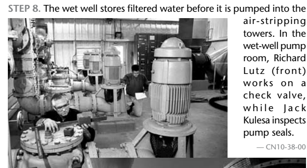
STEP 8. The wet well stores filtered water before it is pumped into the air-stripping towers. In the wet-well pump room, Richard Lutz (front) works on a check valve, while Jack Kulesa inspects pump seals. — CN10-38-00
