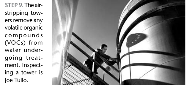
STEP 9. The air-stripping towers remove any volatile organic compounds (VOCs) from water undergoing treatment. Inspecting a tower is Joe Tullo. — D2840306
