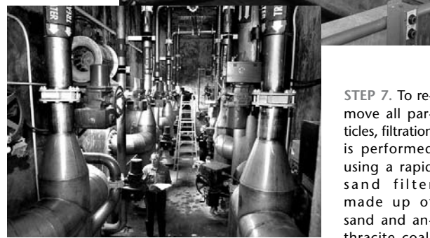
STEP 7. To remove all particles, filtration is performed using a rapid sand filter made up of sand and anthracite coal. Results are reported to the Suffolk County Department of Health Services and to BNL's Environmental & Waste Management Services Division, which ensures that the Lab's water complies with all applicable regulations. — D2750306
