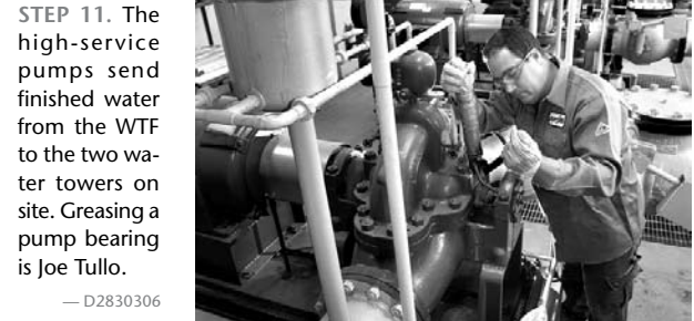
STEP 11. The high-service pumps send finished water from the WTF to the two water towers on site. Greasing a pump bearing is Joe Tullo. — D2830306
