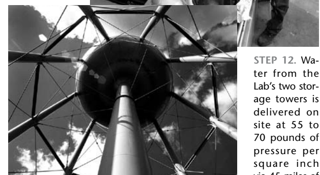
STEP 12. Water from the Lab's two storage towers is delivered on site at 55 to 70 pounds of pressure per square inch via 45 miles of distribution pipe. Viewed from its base is the larger of the Lab's towers, which holds one million gallons of water. — CN10-44-00
