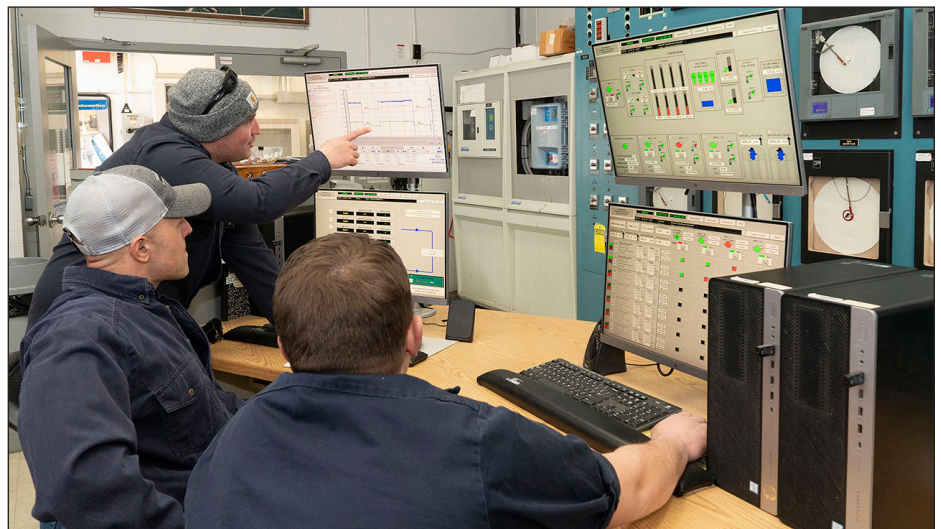
Water treatment operators in the BNL control room reviewing SCADA trend graphs. L-R- R. Kelley, N. Risi, and S. Kelvas
