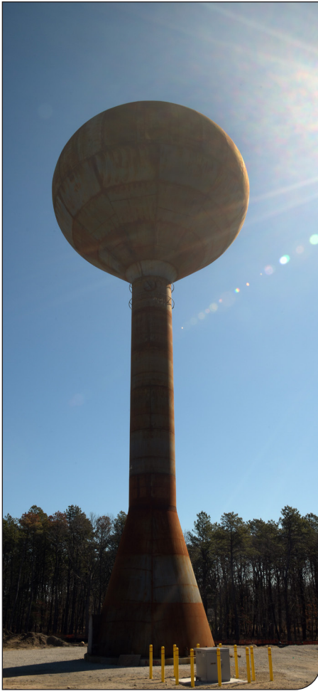
New elevated water storage tank on Upton Rd.
