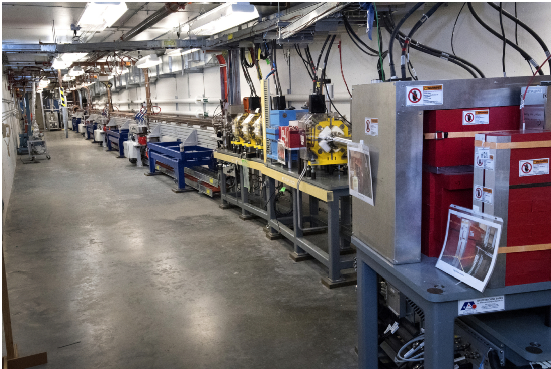
Figure 6.141: NSLS-II pre-injector LINAC.
