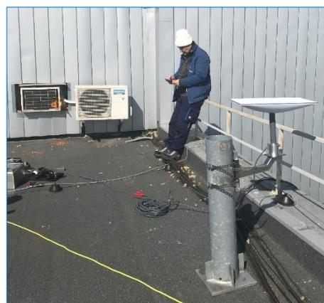
Figure 55: Enhancing the RDT Network: A Starlink satellite antenna was installed in Chernobyl in response to network disruptions caused by Ukrainian mobile network damage in the conflict's early stages (Q1 2022). The depicted Department staff member is setting up the antenna using a mobile app.
