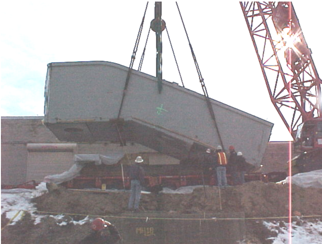
Duct section 4 moments before it rotated (counter-clockwise as viewed) in the rigging (1/29/01).
