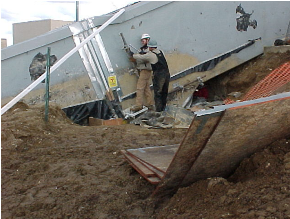
Installation of the diamond-wire-cutting equipment to cut duct section 1N/S support pedestal.
