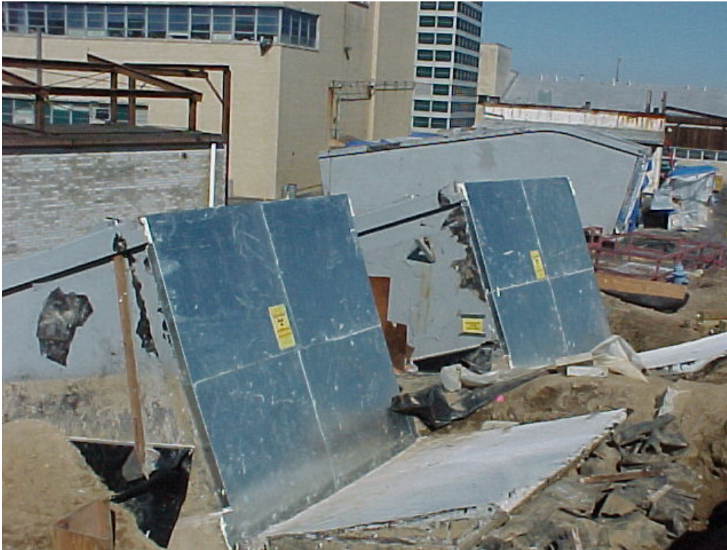
Sheet metal seal covers installed on Below-Ground Duct openings (3/15/01).
