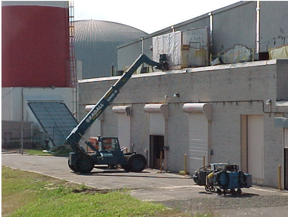
URS workers setting diamond-wire-cutting enclosure on roof of Building 704.
