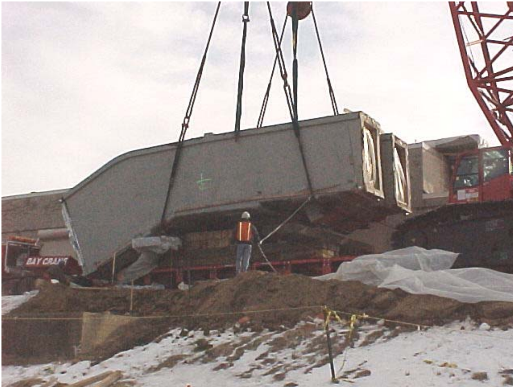
Duct section 4 after it came to rest after shifting in the rigging (1/29/01).
