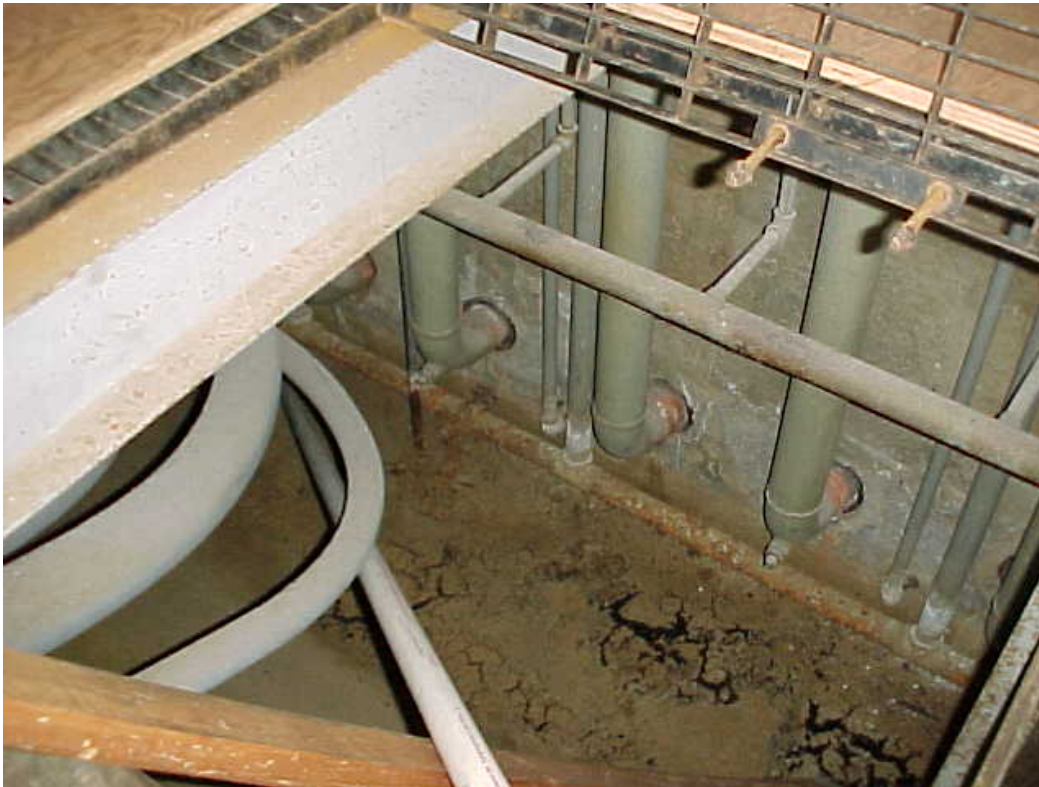
Cooling water penetrations into Below-Ground Duct.
