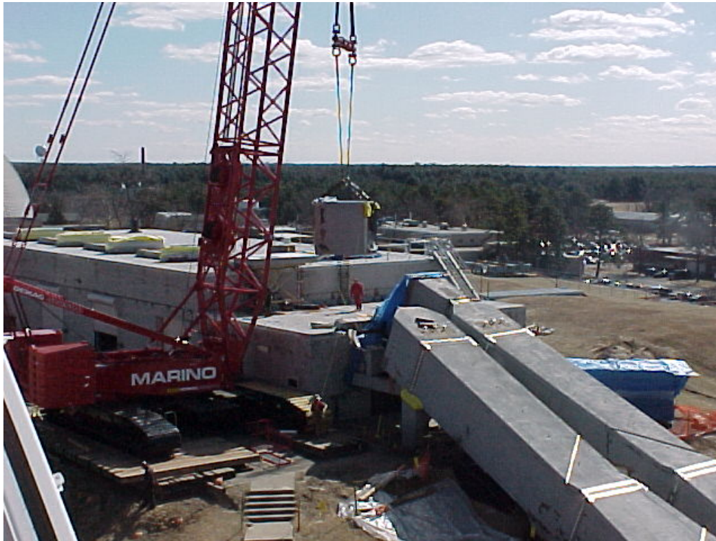
Lifting duct section 3N (2/28/01).
