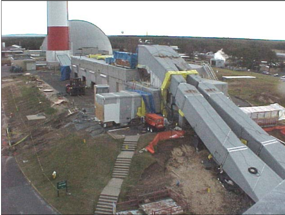
View of duct section 5 being segmented into smaller pieces. The yellow containment for the section 4/3 separation cut is visible.
