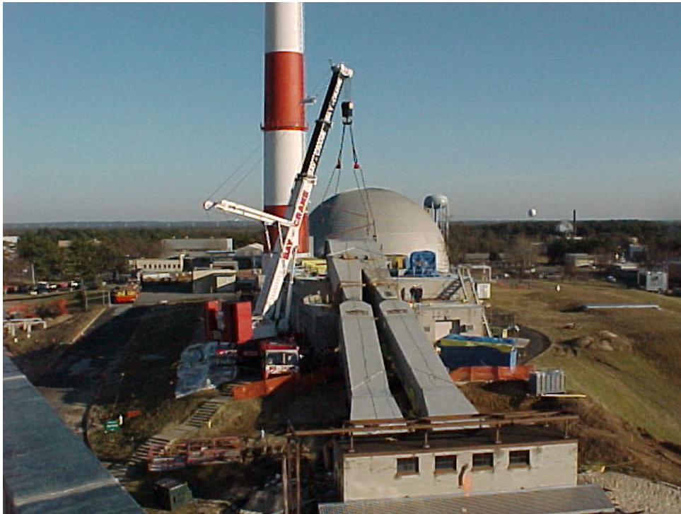
Rigging in place to lift duct section 4 (12/18/00).
