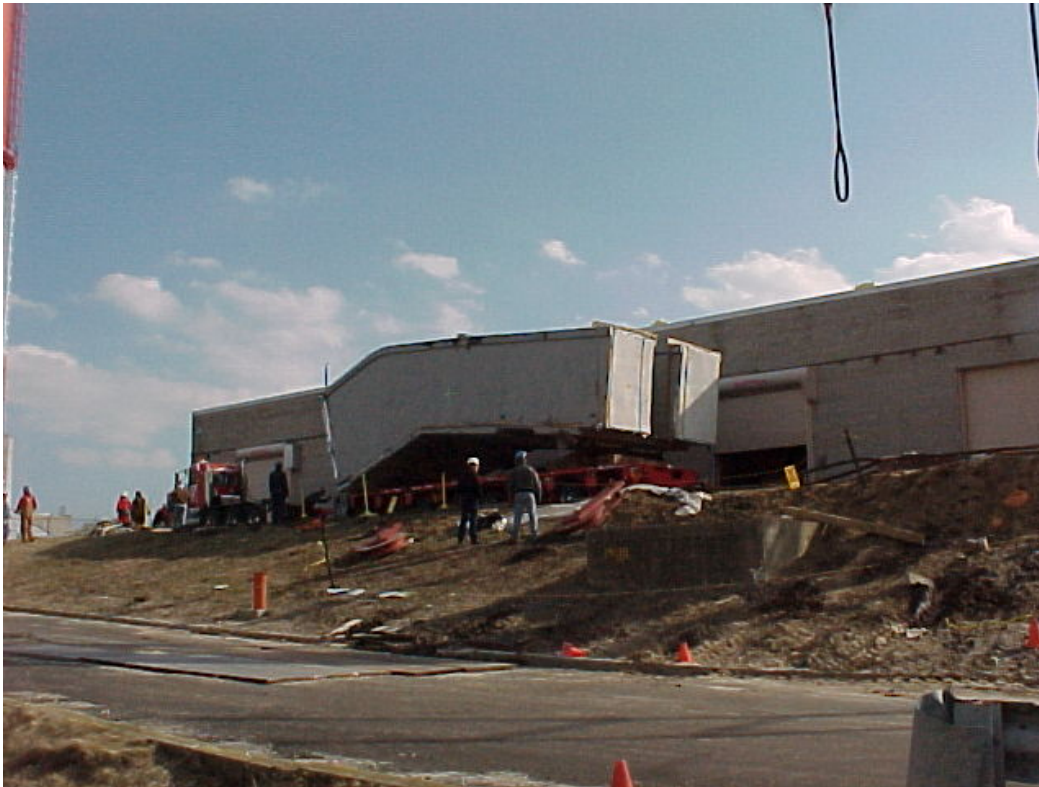
Moving duct section 4 to the laydown area on the Goldhofer trailer (2/27/01).
