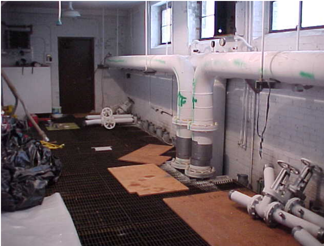
Work in progress - removing cooling water manifolds.
