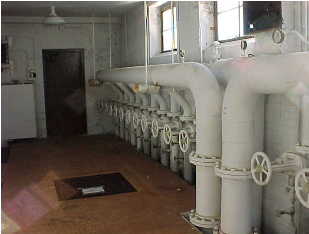
South cooling water manifold.
