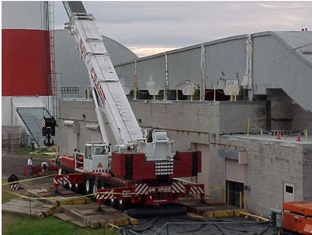
500-ton crane in place to begin lifting duct section 5.
