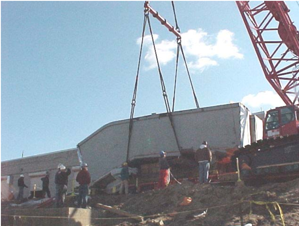
Re-lifting duct section 4 with revised rigging configuration (2/26/01).
