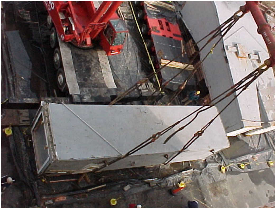
Duct section 1N being lowered onto cribbing (3/3/01).
