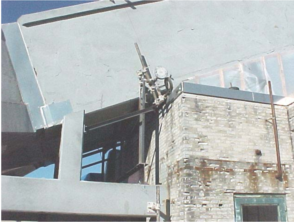
Setting up the diamond-wire-cutting equipment to make the section 4/3 separation cut.
