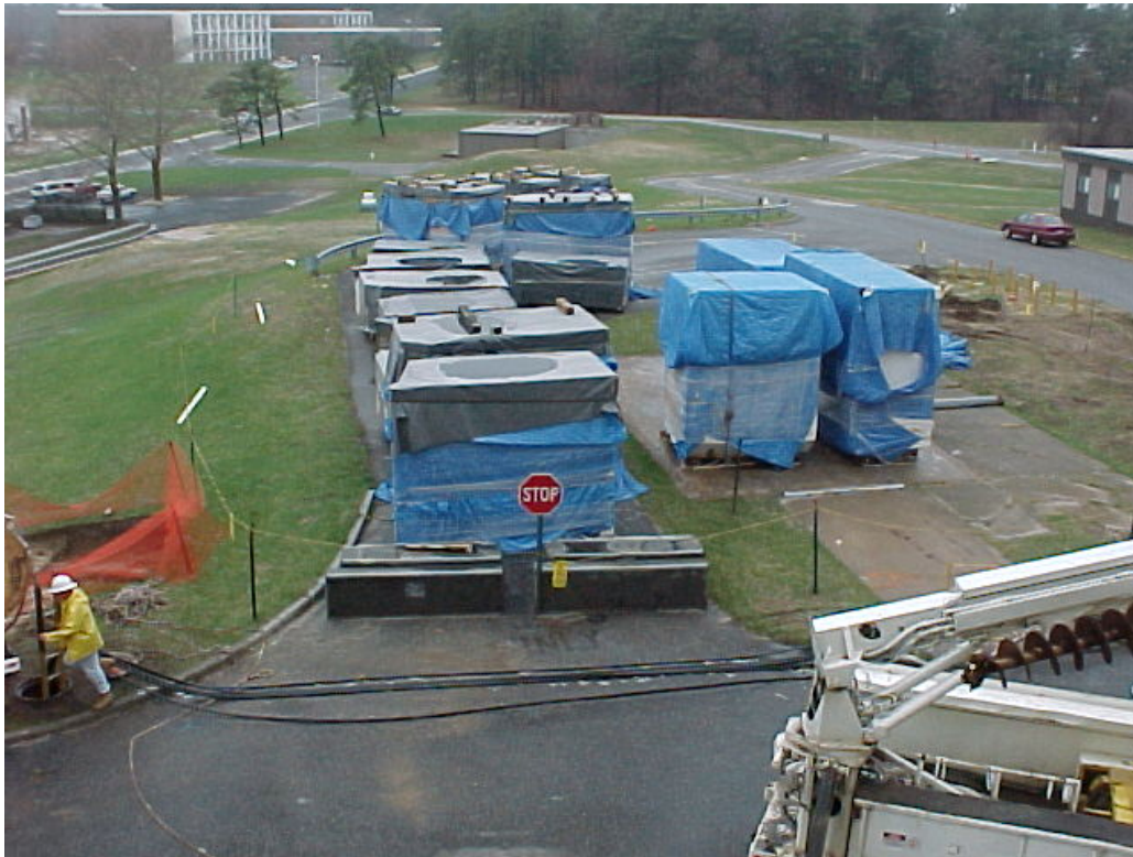
Maintenance and covering of ducts in west side laydown area (4/12/01).
