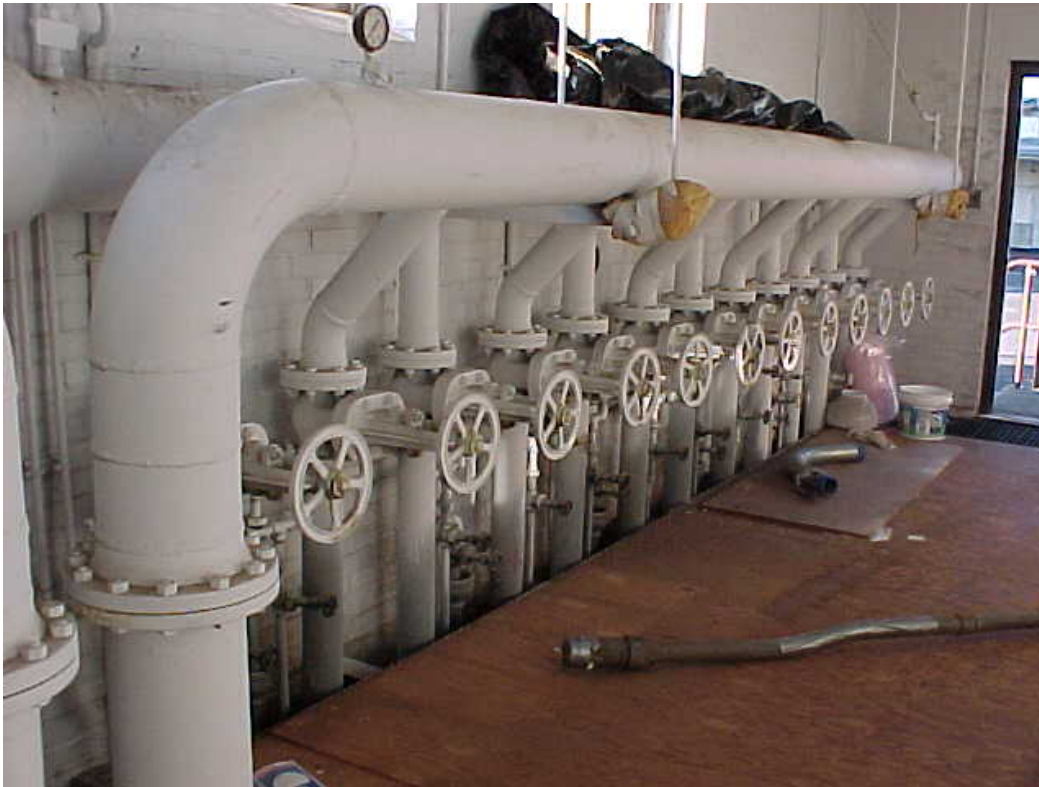
North cooling water manifold.
