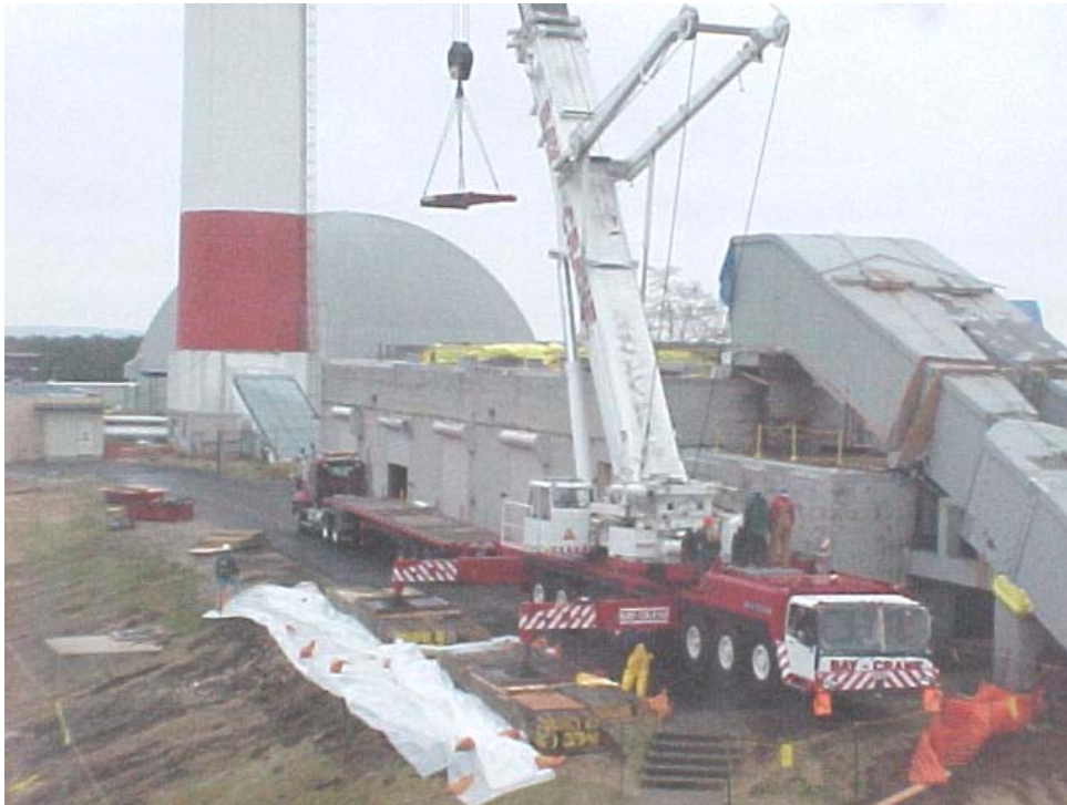
Setting up the 500-ton mobile crane for first lift attempt of duct section 4.
