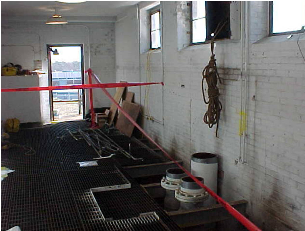
View of West Instrument House wall after removal of the cooling water manifolds. The main supply and return headers are visible at the grating opening.
