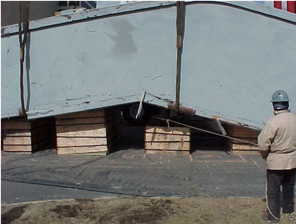
Duct section on the cribbing in the laydown area (3/1/01).
