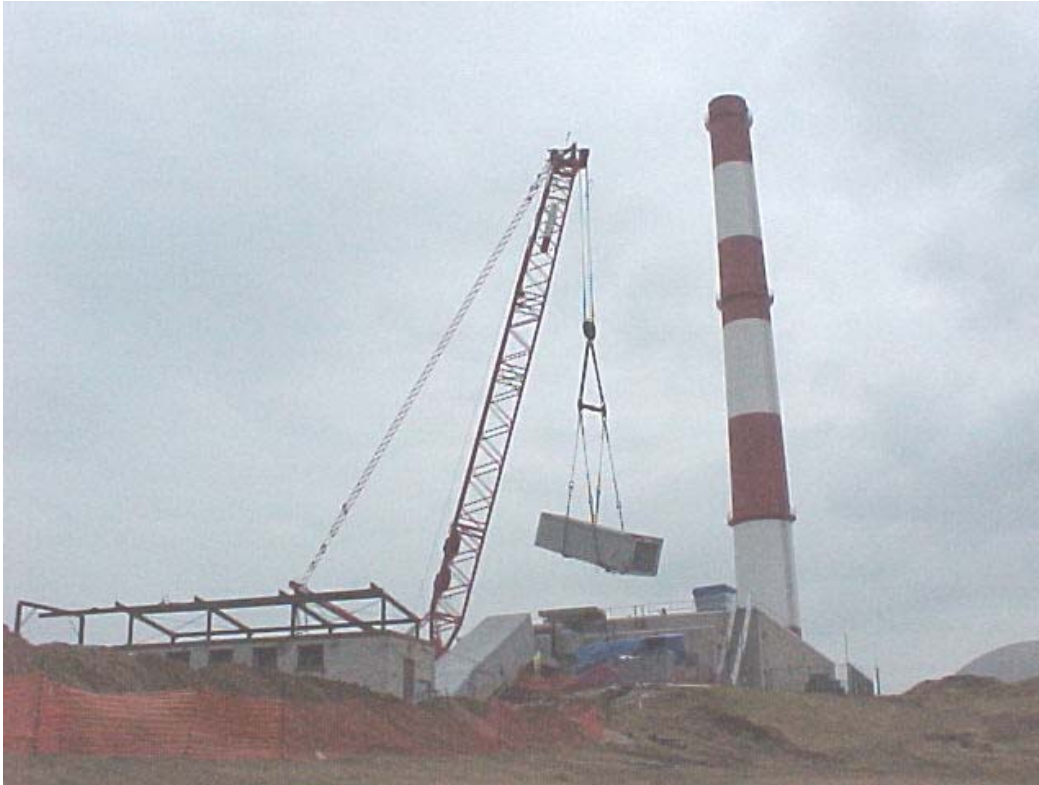
Duct section 1N over Building 704 (3/2/01).
