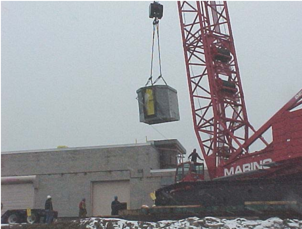
Lifting duct section 2N (3/2/01).
