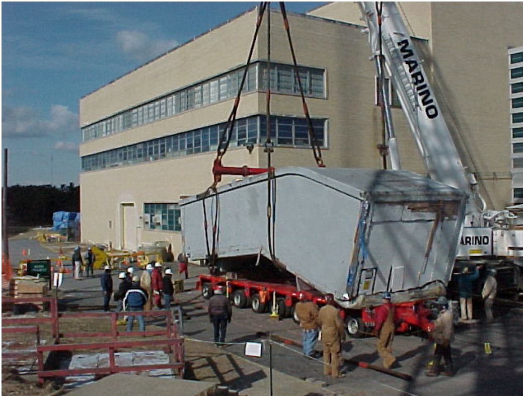
Lifting duct section 4 from the Goldhofer trailer in the laydown area (3/1/01).
