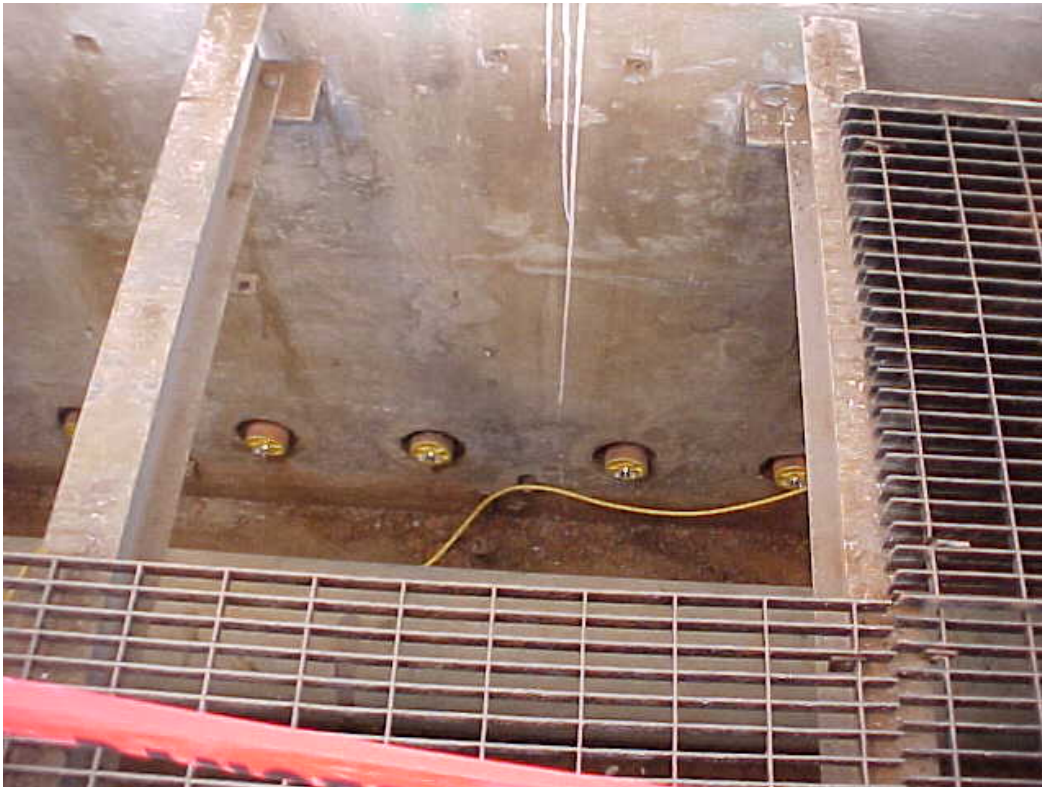
Cooling water penetrations into Below-Ground Duct after being sealed.
