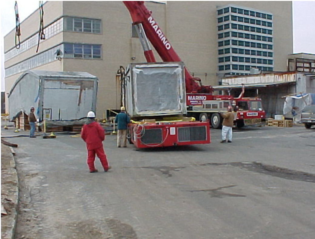
Bringing duct section 1N to the laydown area on the Goldhofer trailer (3/3/01).
