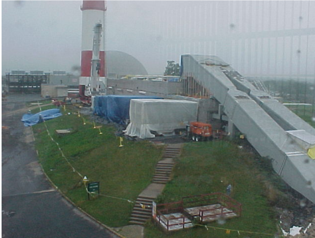
Duct sections 5 through 9 on cribbing after being lifted from roof of Building 704.
