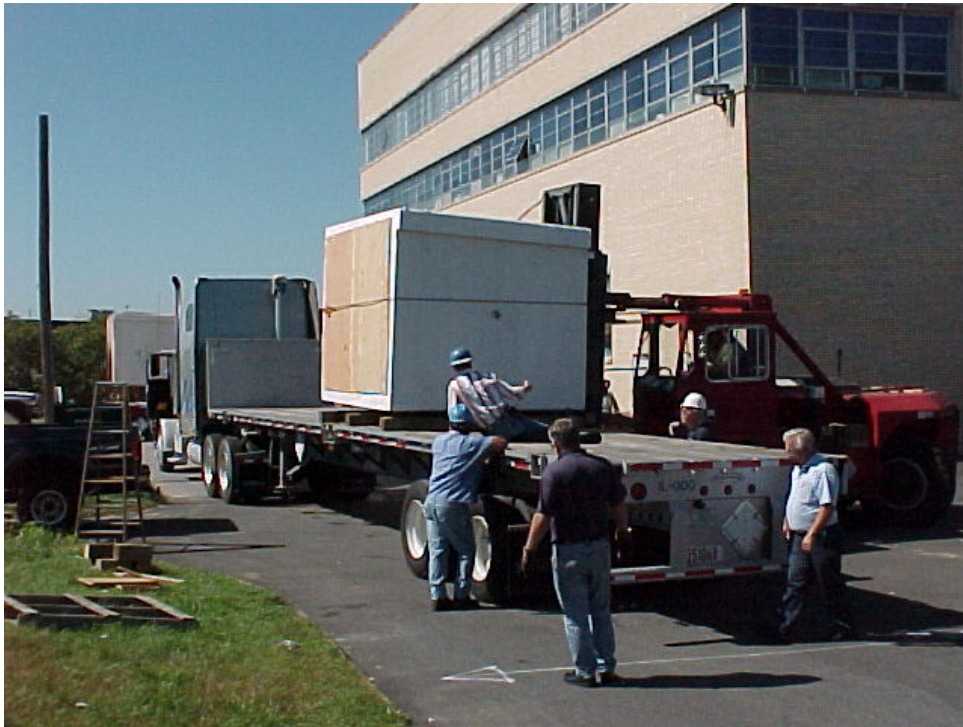
Segmented section of duct being loaded for shipment.
