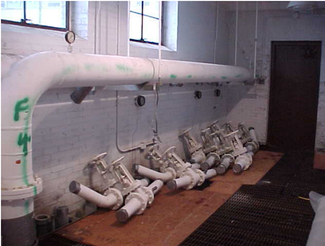
Abandoned valves and piping ready for disposal.
