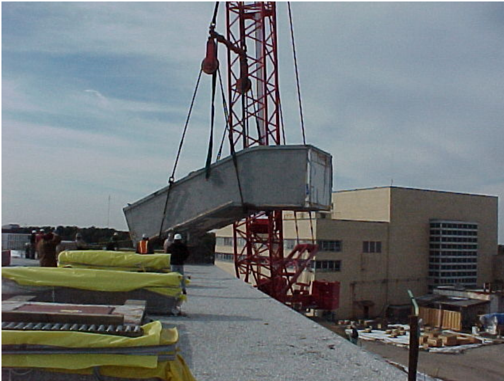
Second lifting of duct section 4 (1/29/01)
