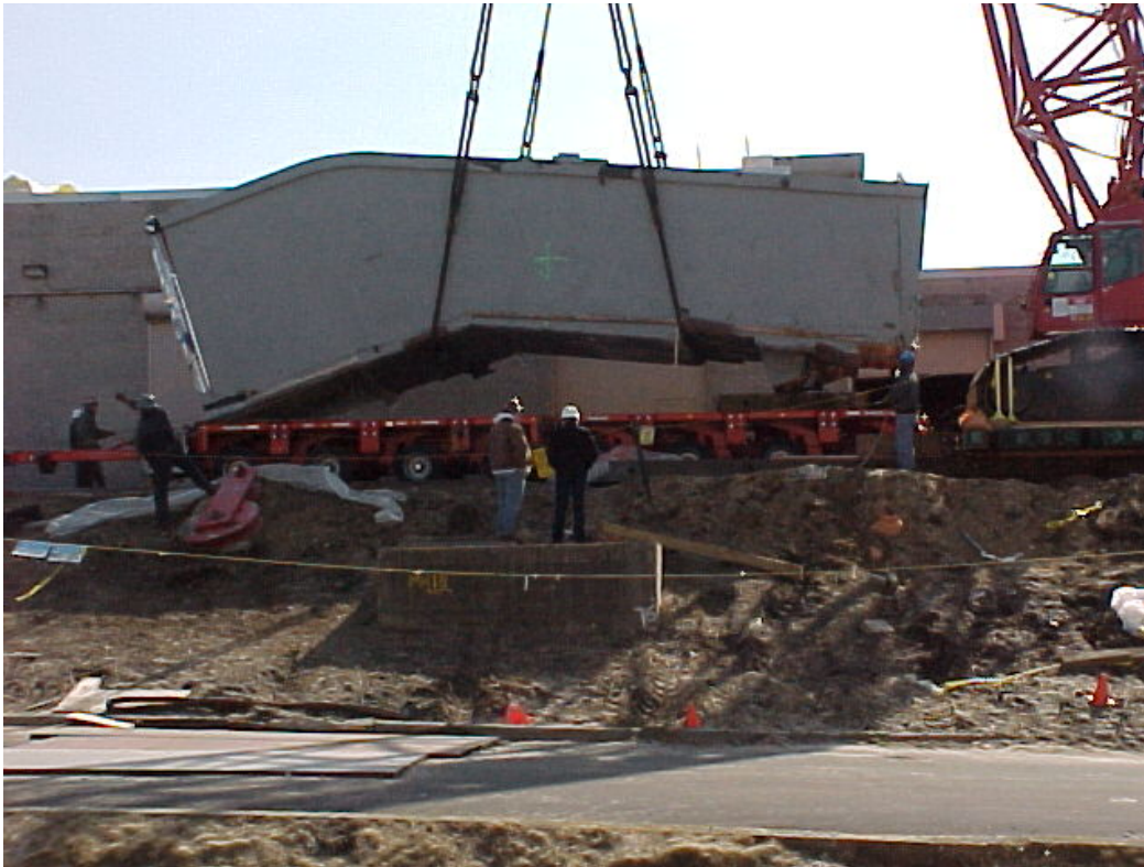
Setting duct section 4 on the repaired Goldhofer trailer (2/27/01).
