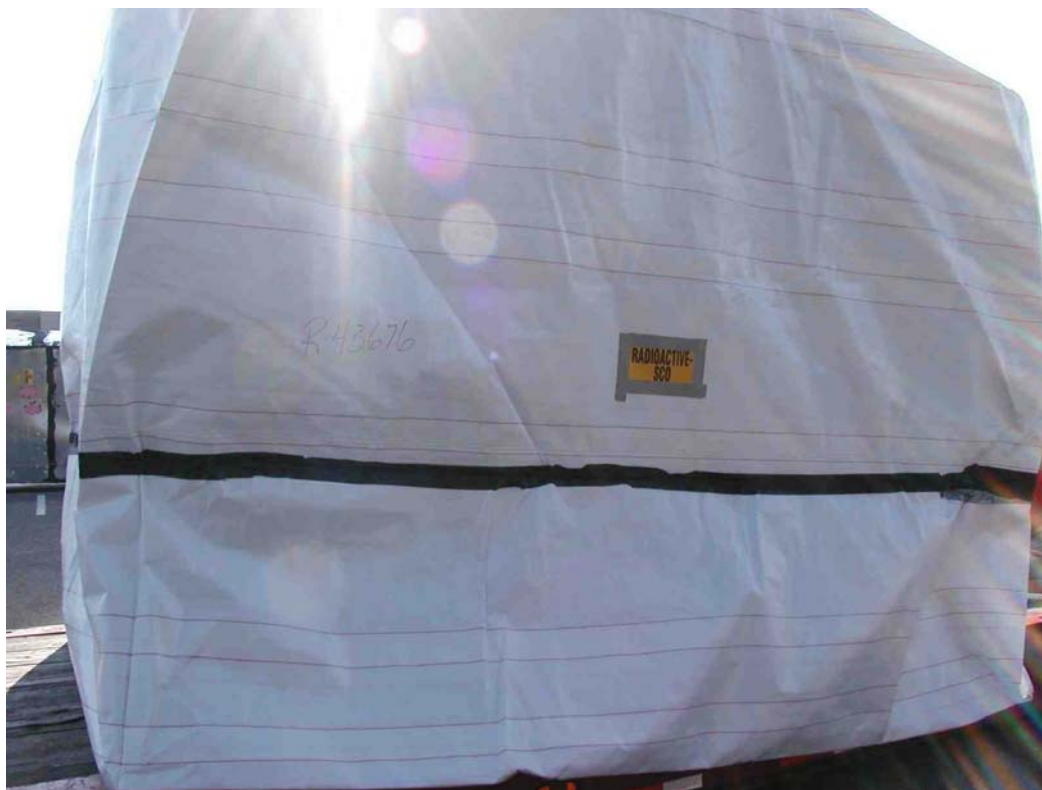
Duct 2S placed in Super Sack.
