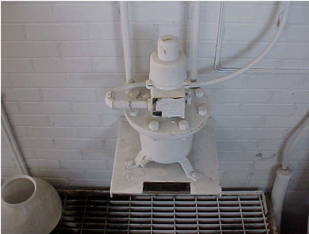
Abandoned flow transmitter
