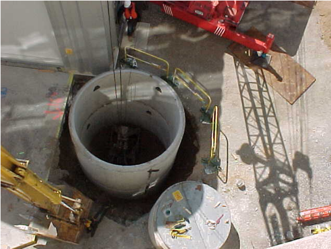
View looking down into the caissons at the below ground duct bustle soil pocket. The excavation process involved removal of soil from within the caisson, and as the soil was removed, the caissons advanced downward. Additional caissons were added as the depth increased.
