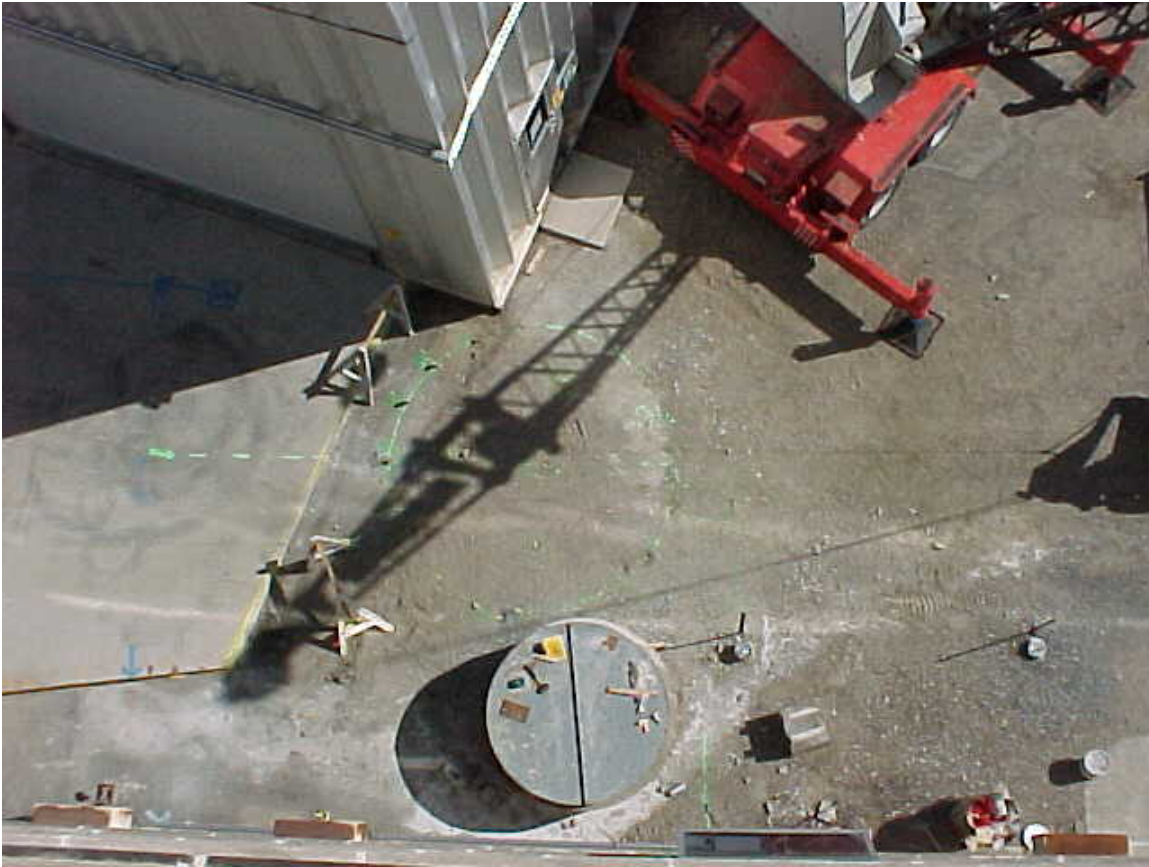
View looking down on the caisson that was used to access the below ground duct bustle soil pocket. The location of the contaminated soil pocket that was located between 27 feet and 30 feet below grade.
