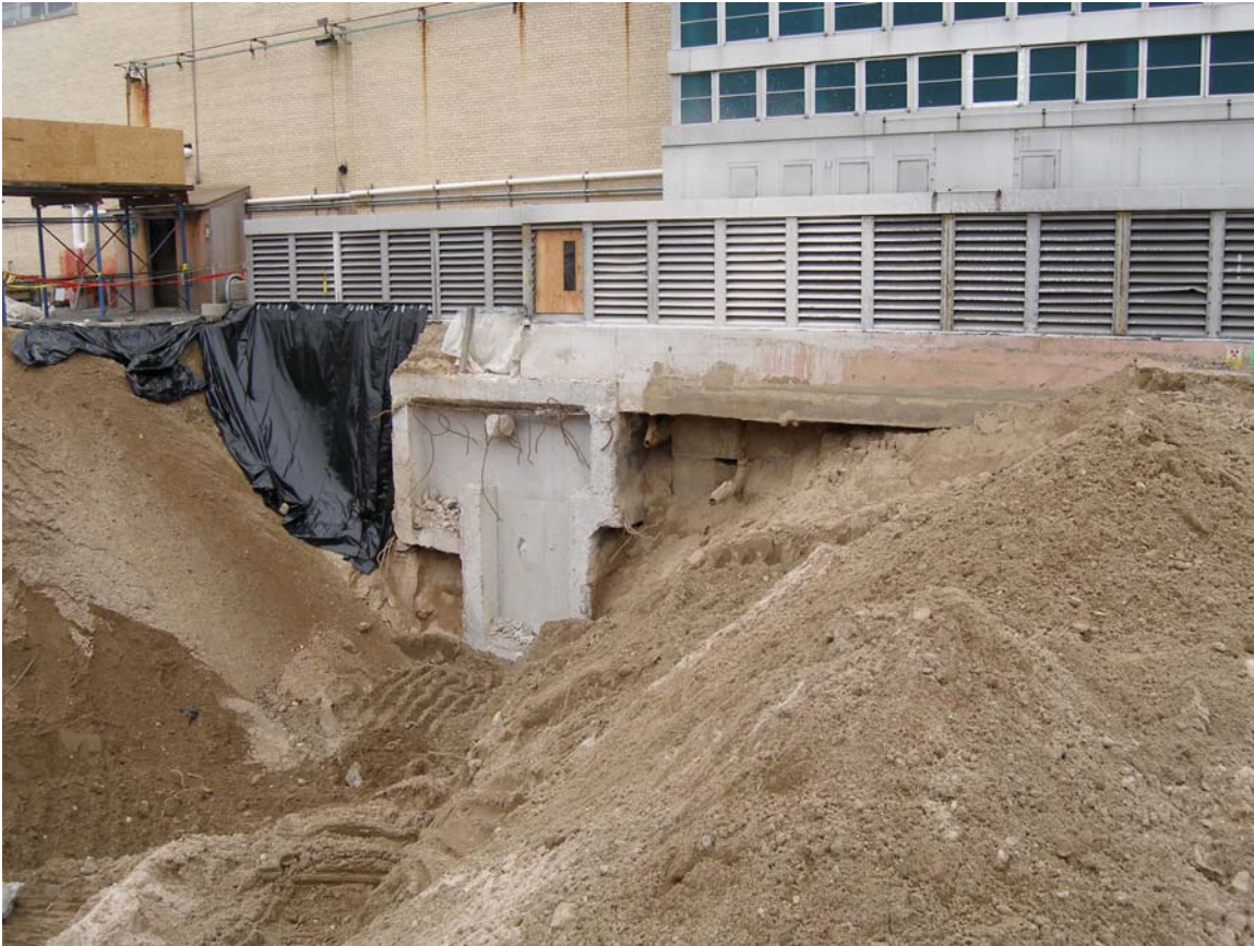
View of the 20" thick reinforced concrete wall constructed at the canal removal point. The cut line of the canal structure is located 4'-3" east of Building 701 column 101. Floor and roof drain lines that had been previously cut and abandoned can be seen hanging beneath the floor of the east intake structure.
