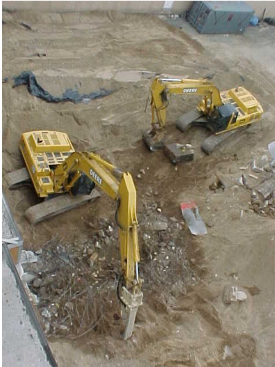
Canal excavation and demolition in progress. Here, one John Deere excavator is being used to demolish the south canal wall while the other is excavation soil.
