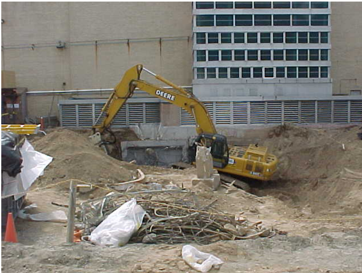
Canal excavation and demolition in progress. In the foreground is the steel rebar from the concrete. At center photo, part of a concrete buttress can be seen. In the background, the top of the canal can be seen at the cut line. The John Deere excavator is being used to demolish the sough canal wall at this time.
