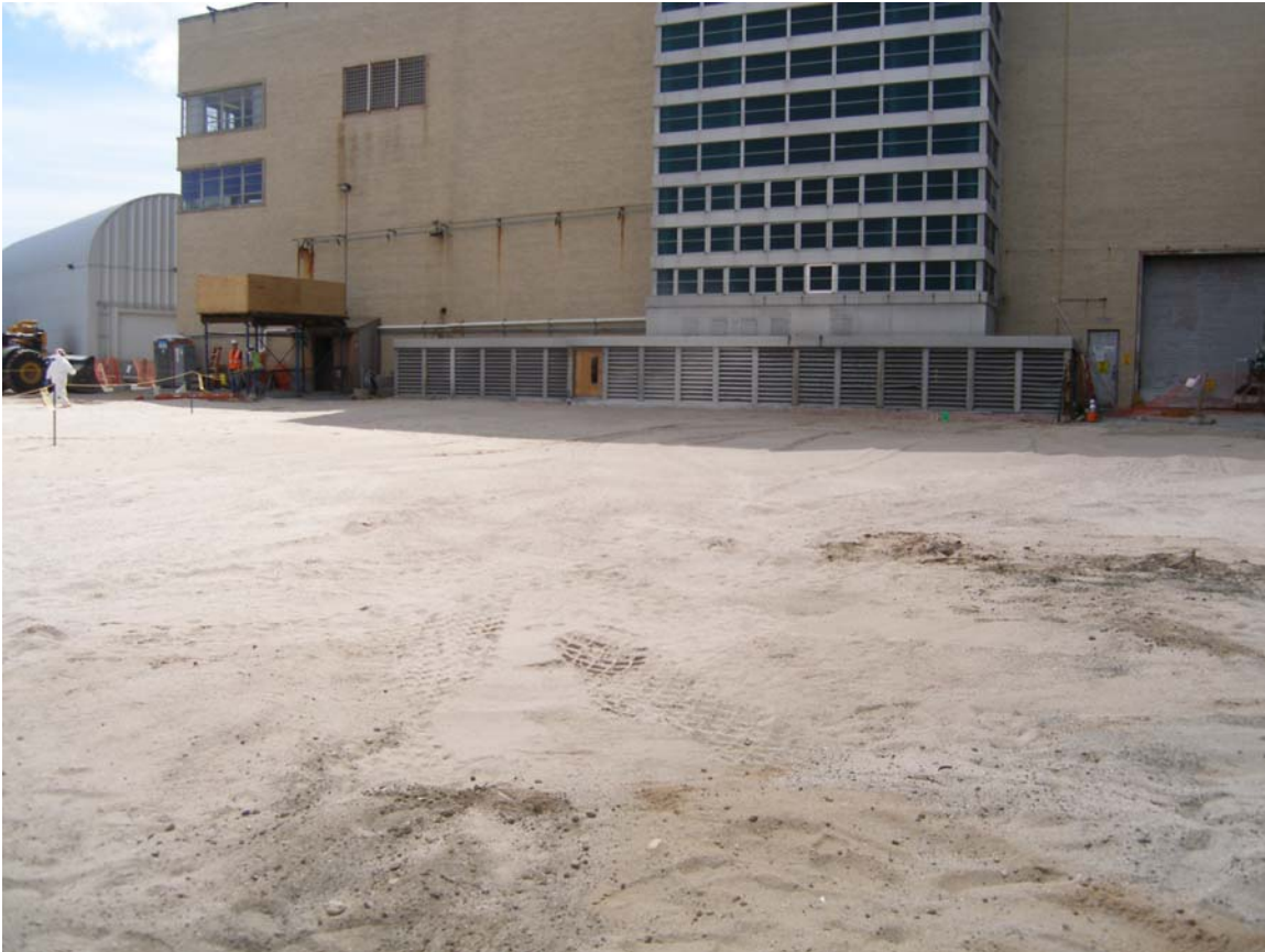
View of the canal excavated area after backfill and compaction to the pre-existing grade.
