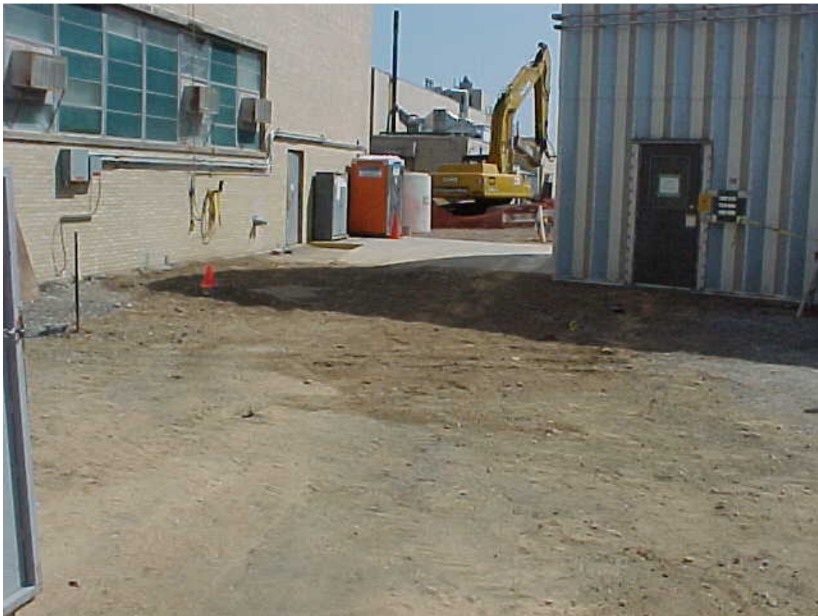
View of the area of the soil pocket removal at the below ground duct bustle after backfill and initial compaction.
