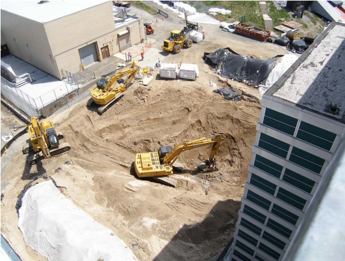
Canal excavation and demolition nearing its end. The John Deere excavator is being used to excavate the last remaining concrete debris and soil. At the top of this picture, the forklift is carrying a MHF Waste Liner® to the staging area. Two empty liners can be seen staged and ready for filling.
