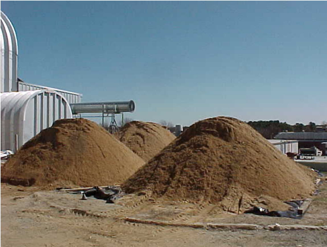
View of the clean overburden soil that was removed from the below ground bustle area above the known location of the contaminated soils that were located between 27' and 33' below grade.
