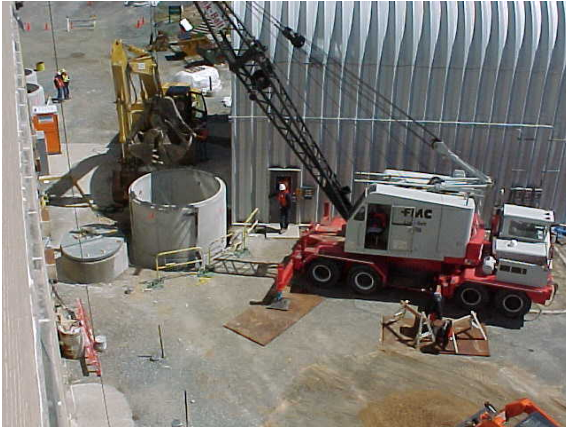
Installation of the third of four concrete caissons at the below ground duct bustle soil pocket.
