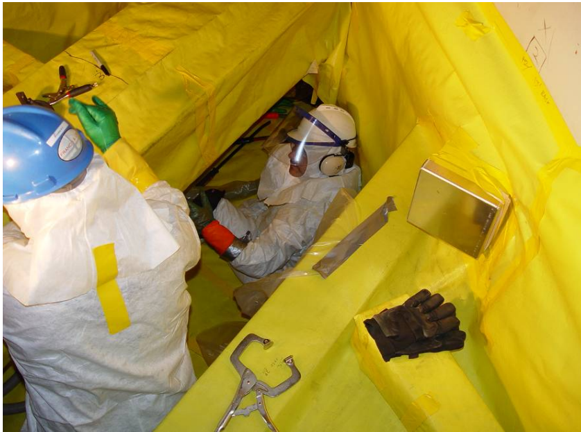
Photo 1 Control Rod Cutting and Removal
