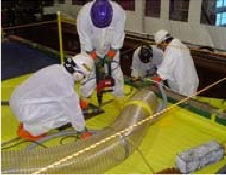
Photo 2 Boron Shot Removal
