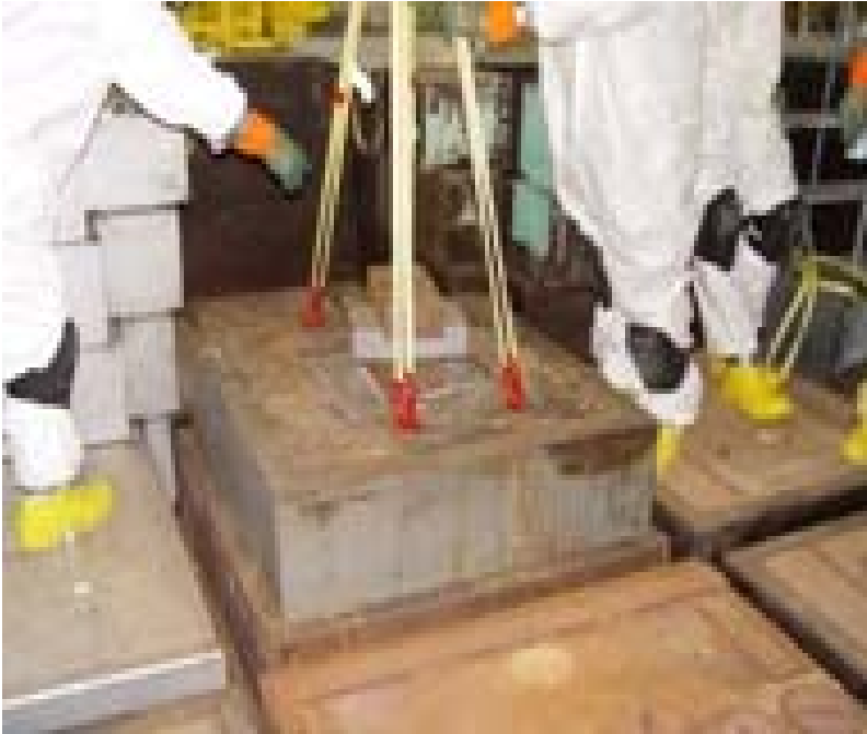
Photo 3 Roof Plug Removal
