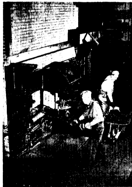
James Carter stirs coals while Matnew Campanaro fuels the automatic stoker. In background Joseph Ferlitto tends the reserve boiler. 11 men work on three shifts keeping the pressure at 375 tons for the hospital and apartment area. These giant boilers use 20 tons of coal per day. Four big heating plants and 13 small units keep a crew of 44 men busy day and night.
