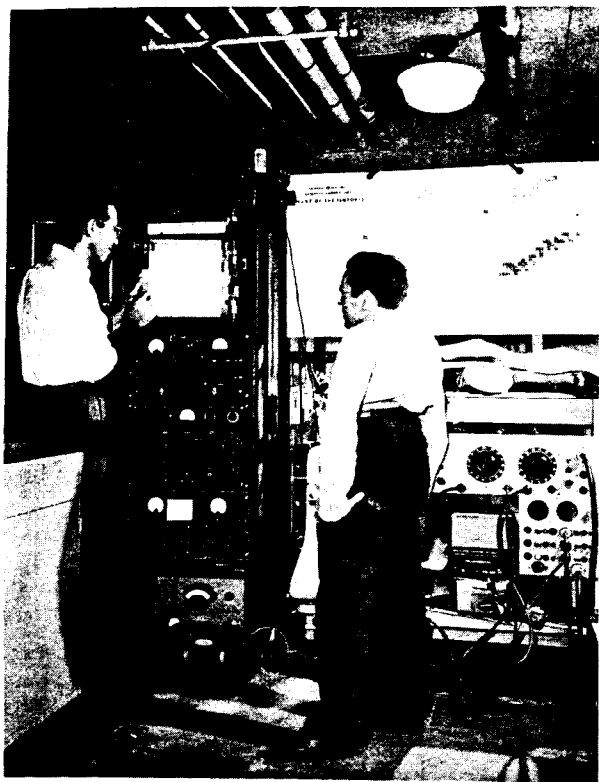
Dr. Julius Hastings and Dr. Oliver Schaeffer operating a mass spectrometer to study the forces which hold molecules together.
