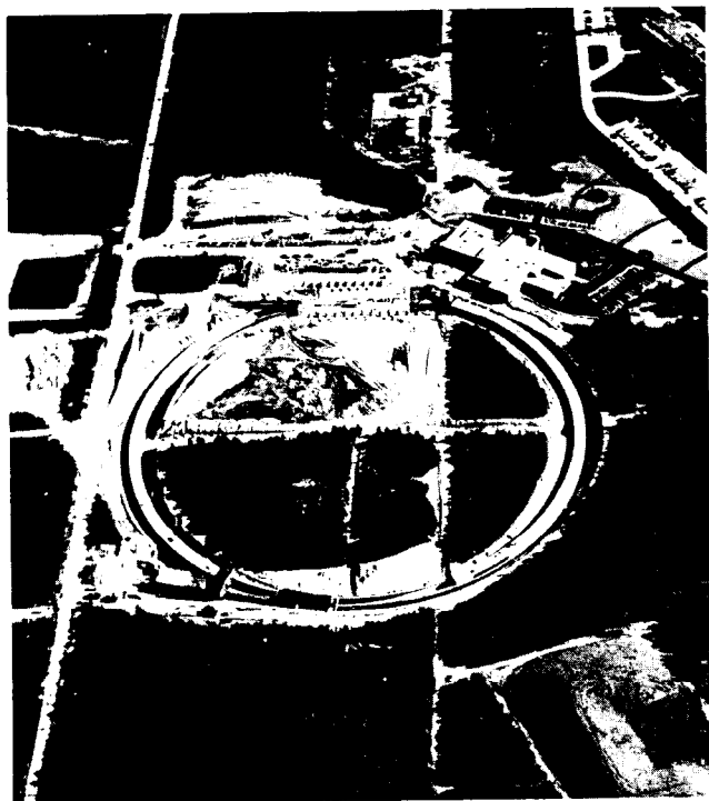
Construction of the AGS - photo taken in 1956.
