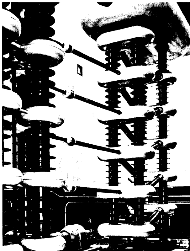
Cockcroft-Walton Generator soon after installation in 1959. This machine provides the initial acceleration to the protons, after which they are injected into a linear accelerator before entering the orbit of the AGS.
