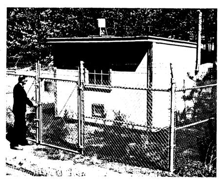
The most conspicuous aspect of this area survey program is the nine Area Survey Stations, one of which is pictured above. Three of the stations are located on-site, four are at or near the perimeter, and two are off-site. Sensitive Dynamic Condenser Electrometer Ion Chamber units within these stations
