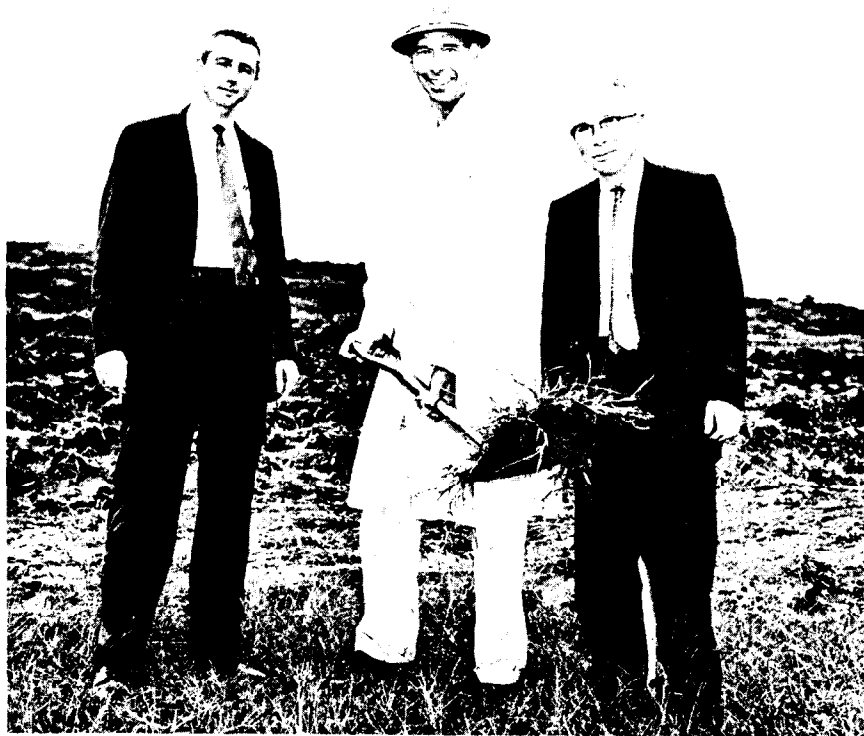
Clarke Williams, Nuclear Engineering Department Chairman taking the first shovelful of earth, with Joe Hendrie, Project Engineer and Thomas Sheehan, Project Manager of the HFBR.
