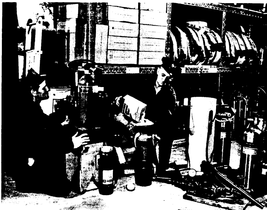
Ed Yost (left) weighs a carbon dioxide fire extinguisher to determine whether the unit needs to be recharged. Walter Ceberek recharges a dry chemical extinguisher. Each of the 1742 extinguishers on site is checked about four times a year.
