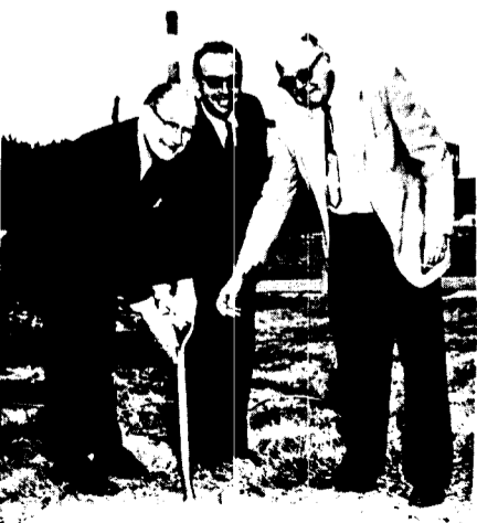
SPADEWORK - Dr. T. Keith Glennan (left), President of AUI, Dr. Maurice Goldhaber, Lab Director, and Mr. Donald Moore (right), Director of Engineering and Construction of the Brookhaven Office of the AEC, begin the construction for the new Lecture Hall-Cafeteria Building. Photo by Bob Walton
