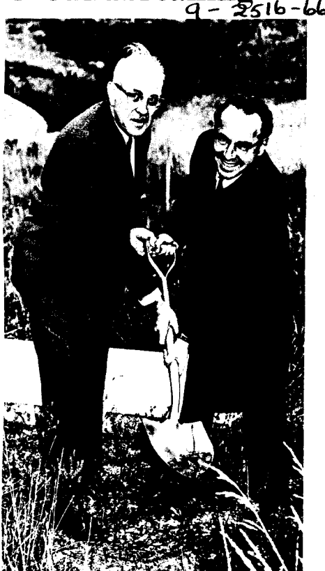
THE BUILDING - Emery L. Van Horn (left), Manager of the Brookhaven AEC Office, and Dr. Maurice Goldhaber, BNL's Director, turn over a spadeful of earth to start the construction of the building to house the Tandem Van de Graaff accelerator system. The building will be completed by 1968; the accelerator system in operation by 1970.
