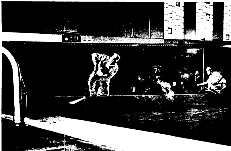
Painters from the Building Maintenance Section of Plant Engineering and Planning are shown putting the finishing touches on the paint job at the BNL swimming pool. The new windows in the background were also part of the refinishing job at the pool that will be completed this week.
