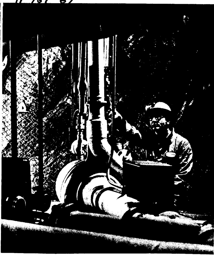
Morris Perlman in pump room. Chain-link fencing bolted to walls and ceilings prevents rock fragments from falling.
