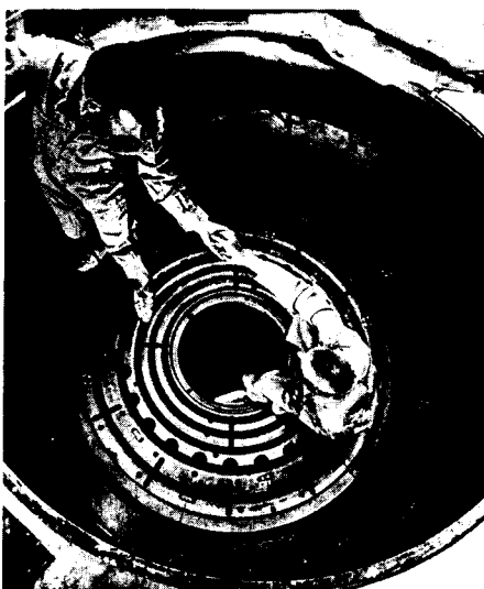
The fuel element hole spacing of UHTREX (Ultra High Temperature Reactor Experiment) at the Los Alamos Scientific Laboratory was carefully checked during core assembly.
