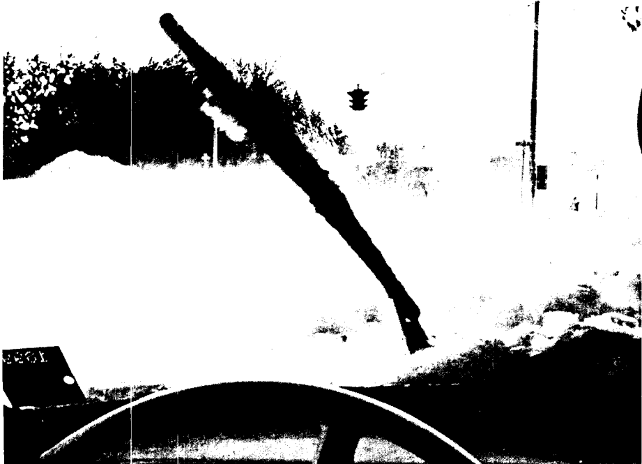
Bulldozer working at the corner of Brookhaven Avenue and Upton Road works amidst blowing snow early on Monday morning. Photo by Humphrey
