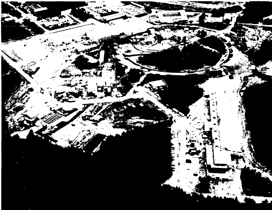
Modification work in progress at the AGS includes: 200 MeV Linac complex (lower right) with earth shielding covering the Linac tunnel to right of the Equipment Bay. Directly above can be seen a section of the AGS ring that has had additional earth shielding placed above it. Inside the ring are the Motor Generator Power Supply building and the RF Power Supply building. At left top is the new East Experimental Building, large enough to cover a football field. Fifth Avenue (from upper left to lower right) has been routed around newly constructed buildings.
