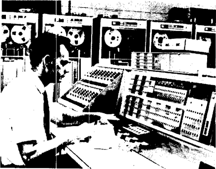
Computer Control Console
