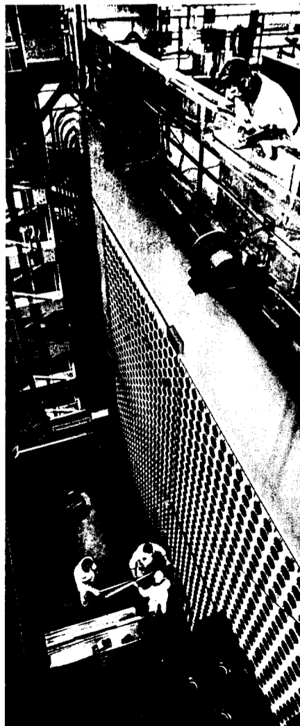
Danny Oldham stands on top of reactor monitoring removal of fuel elements.
