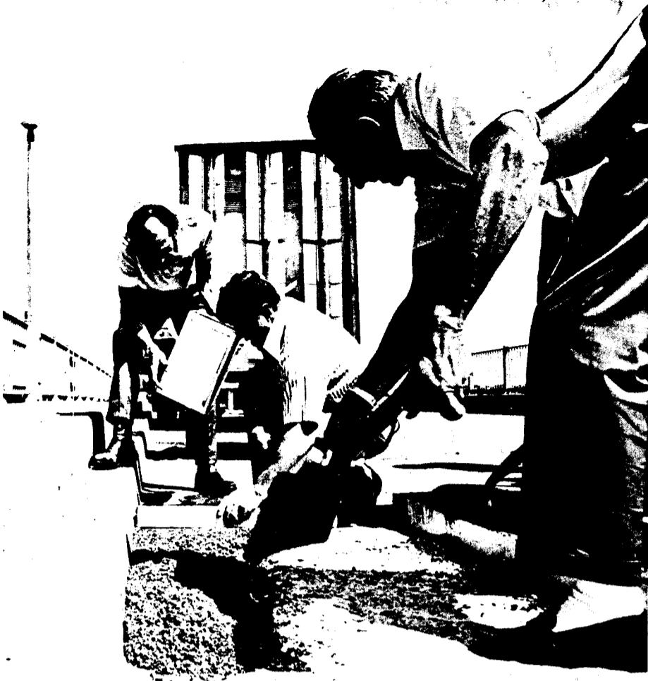
Gus Arnold, Jules Varela and Henry Ruge work together to put a concrete polymer overlay on a bridge pot hole.
