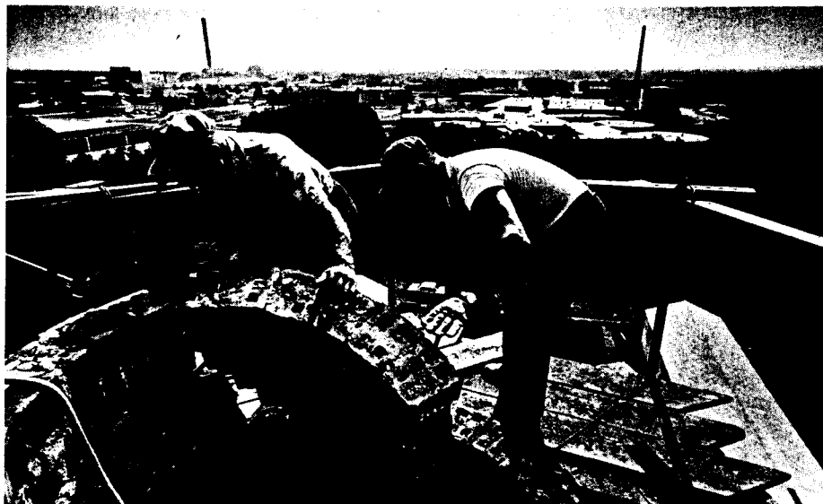
Workmen from the American Chimney Corporation dismantle sections of a stack from one of the laboratory's former steam plants. After the brick and mortar are loosened, the rubble is dumped down the center of the 90-foot chimney, where it is removed through a large hole broken through the base.
