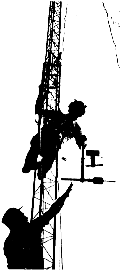
Gil Raynor (bottom) hands an anemometer to John McNeil which he will attach to the tower.
