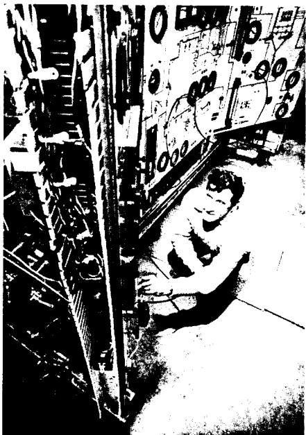
Arnold Roesch inspects the gas purification and re-cycling facility which circulates gas in the spark chambers.
