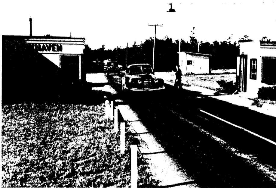
Not a very familiar scene today, but back in 1947 this was the main entrance to Brookhaven National Laboratory.
