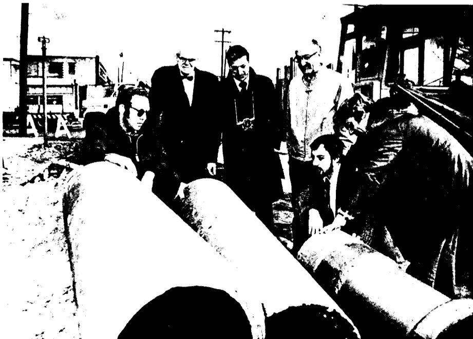
Inspecting the pipes before they are installed are (from left) Barry Galen, Bureau of Mines officials Howard Heginbathan and Harry Makar, Robert Rayfiel from Teledyne, Gary Liss, Principal Engineer, City of Newark and Jack Fontana.
