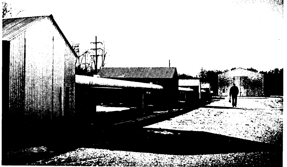
Cryogenic enclosure for superconducting cable stretches across the Fifth Avenue site.
