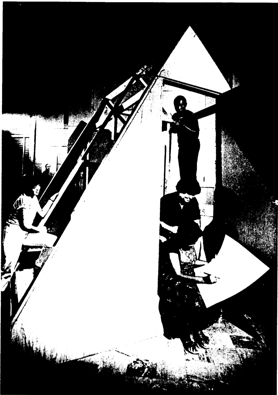
Students in a BNL apprenticeship program assembled the framework for a solar hydroponic greenhouse, which they finished building at the end of their summer term last week. With solar assistance, it can grow enough produce to feed a family of four year-round.
