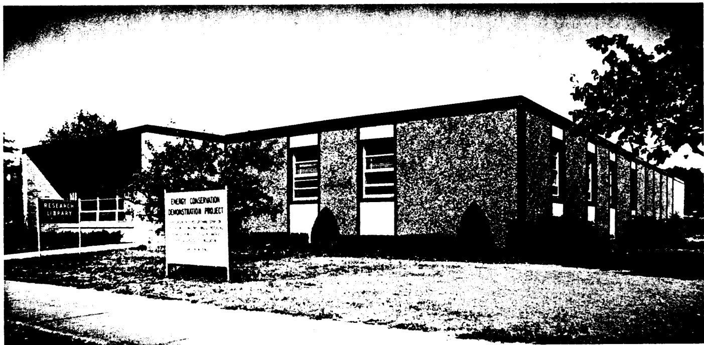
The new look for the Library combines eye appeal with energy conserving ideas. Recently coated with exterior insulation, the south and east walls now have an R value of 17.
