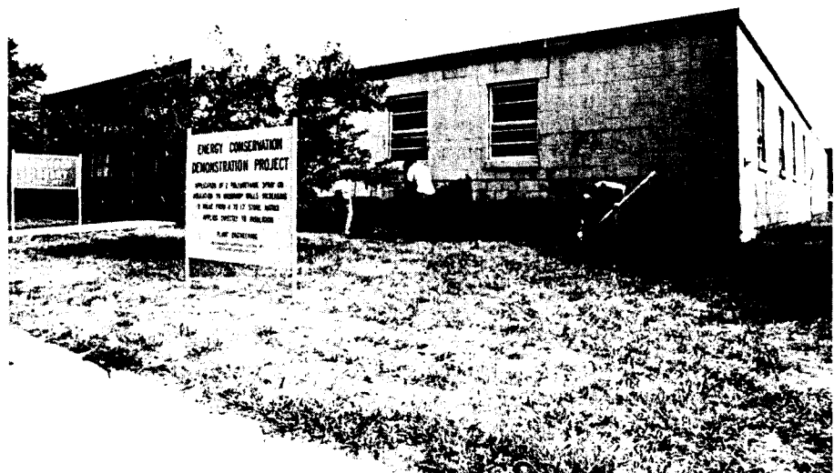
Parts of the old Library exterior showed cracking cinder block walls.
