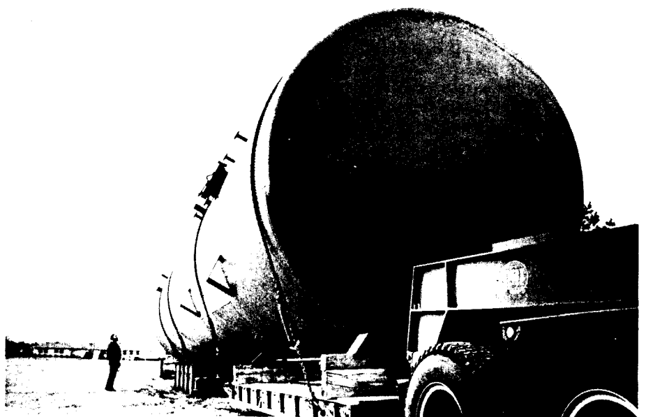
Sixty-thousand gallon tank for ALF delivered to Lab on a 100-foot flat bed truck.
