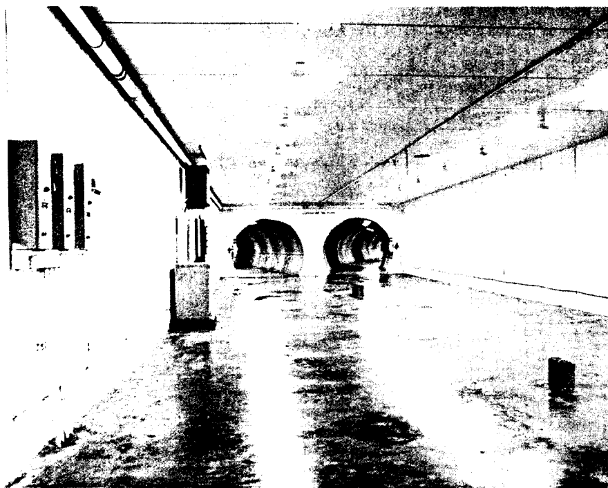
About 98% finished is the South Injection Transition Section. As part of the injection system for ISABELLE, this is the point at which the pipe carrying the beam lines splits into two, in order to inject each of ISABELLE's rings separately. With the completion of the Service Building at the end of this year, the majority of the conventional facilities for ISABELLE will have been finished.
